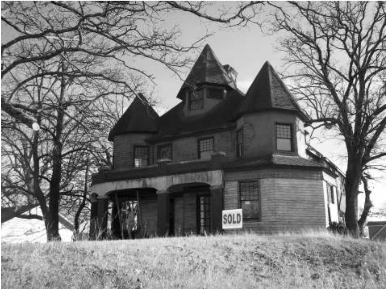
Figure 5: Photo of house prior to restoration.
