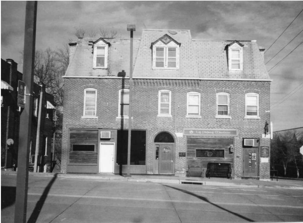
Figure 9. South façade showing central portion and east and west portion
