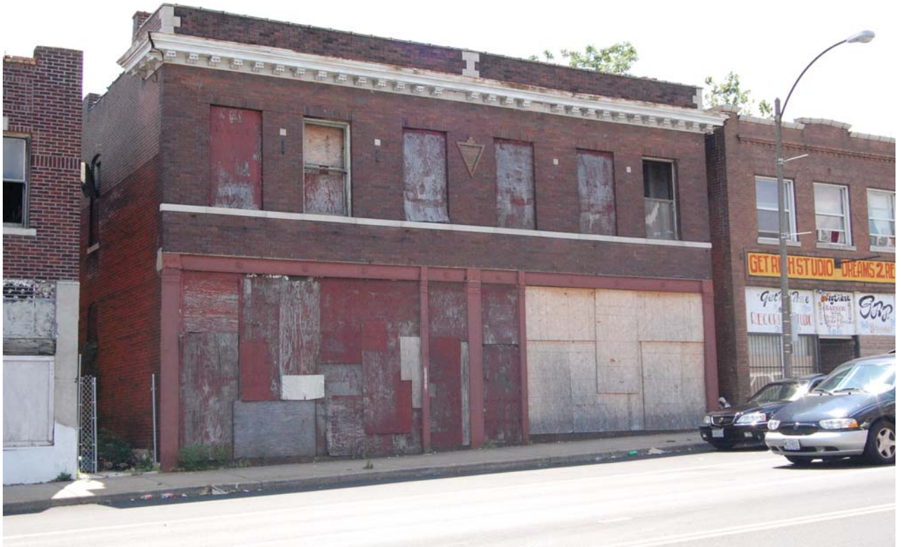
Figure 6. 5806-08 Easton Avenue (Dr. Martin Luther King Drive). The building was constructed in 1909 for a Jewish tailor, Louis Silberstein, who resided upstairs in one of the apartments with his wife, Gussie.
