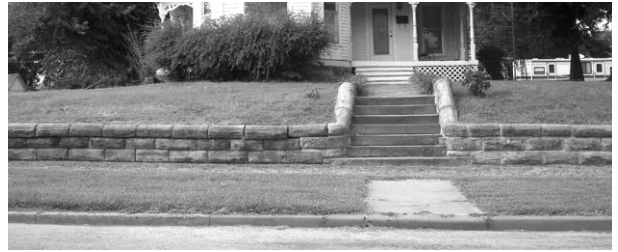
Typical Stone Retaining Wall Found in Phase I Area
