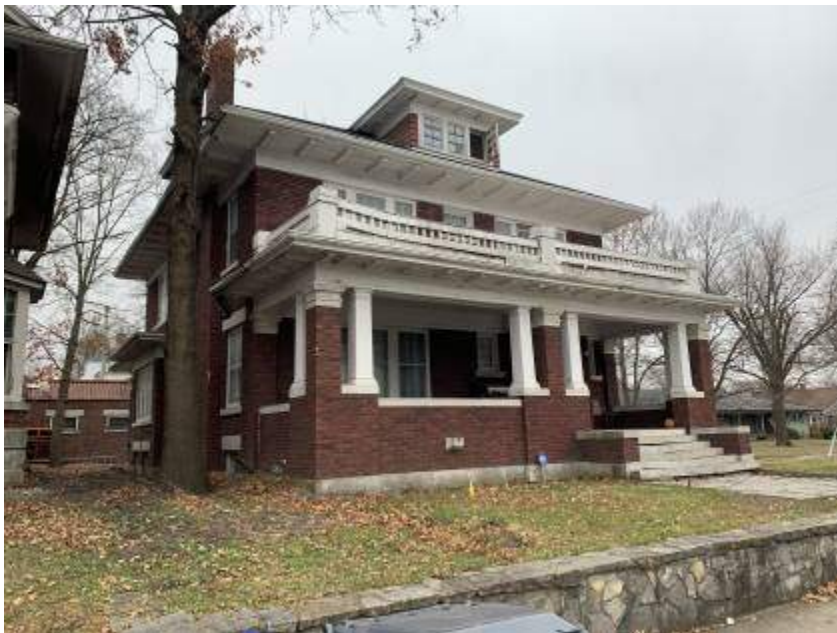
Image 51 – This example could transition as a Colonial Revival style. The Prairie School style was selected, however, due to the wide overhanging eaves and emphasis on horizontality.
