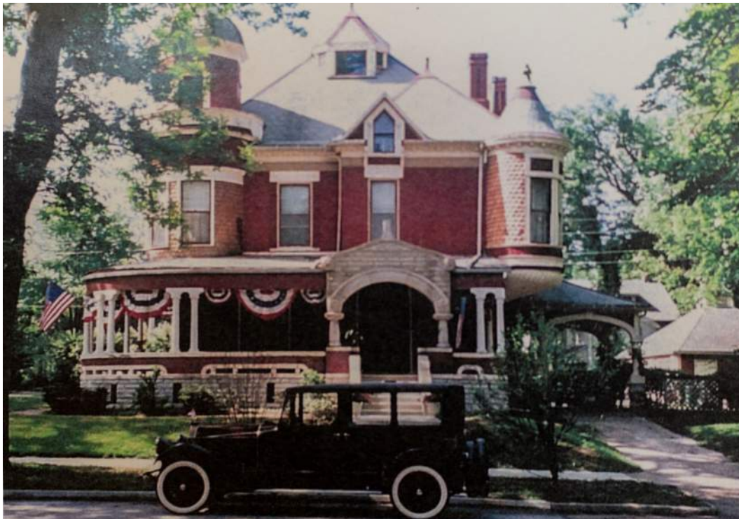
Image 56 – Harris House at 705 W 6 th Street (Source: City of Sedalia, Date Unknown)
