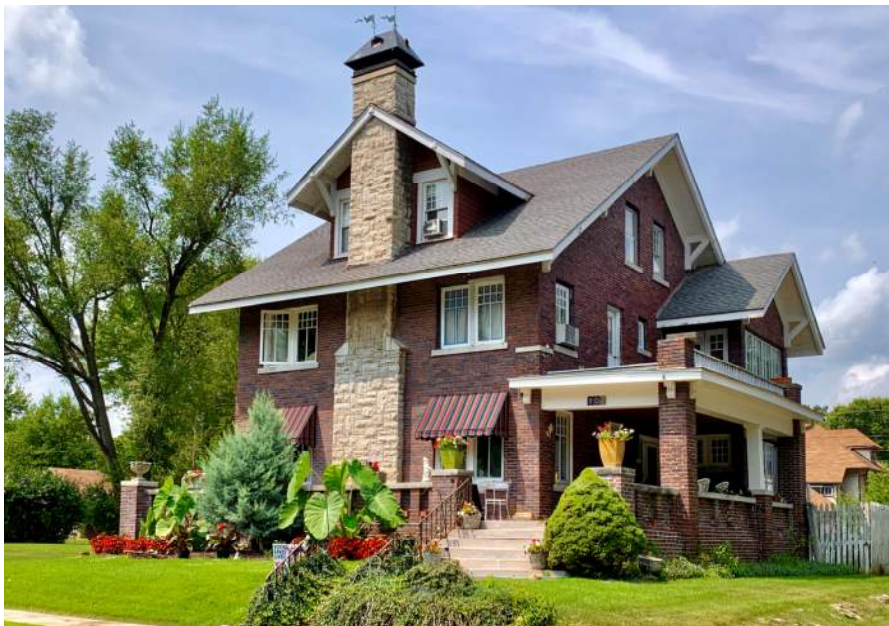
Image 40 – This dwelling on Fifth Street is the best example of the Craftsman Style in the district. It features brick cladding, an unusually centrally placed stone-clad chimney and a side gabled roof with exposed braces.
