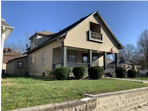
Image 13 – 609 S Park Avenue (West Side of District)
