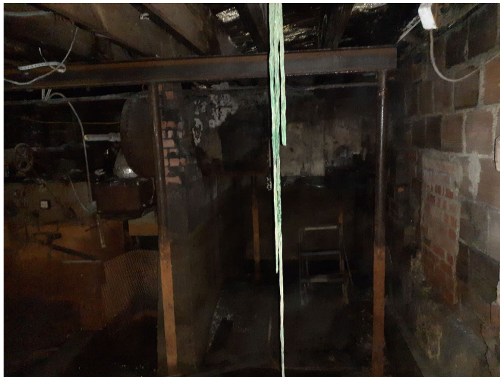
Figure 23: Basement (Former Dressing Room), facing north
