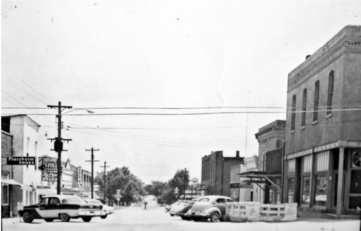
Fig. 3 This 1950s view of South Smith Street looks southward from West Washington Boulevard and shows the People's Bank/Masonic Hall on the right corner. [Crawford County Historical Society]
