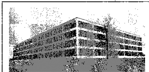
1968-1971 Low-Rise TWA Administrative Office Building
