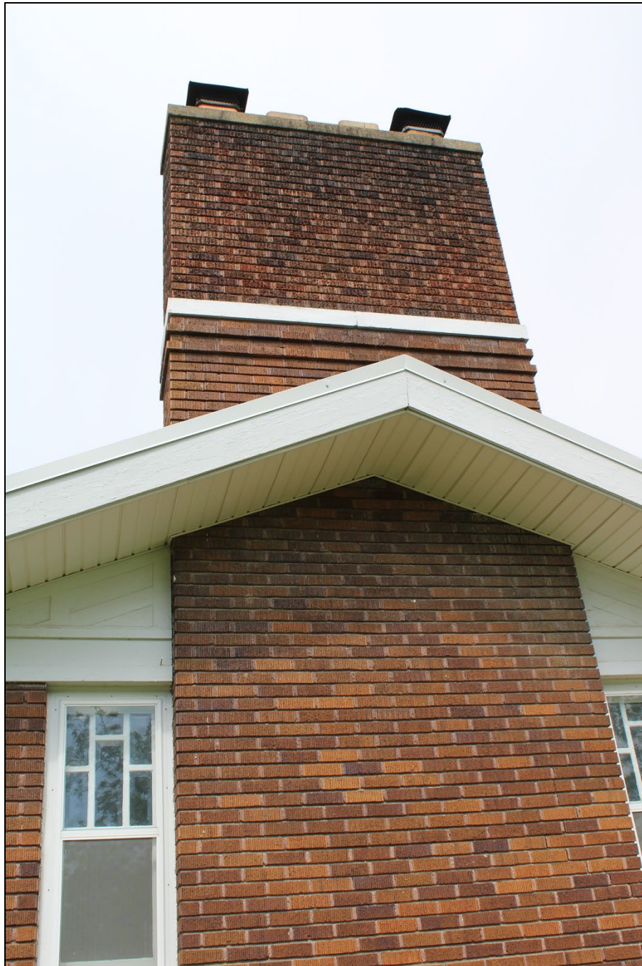
Figure 10: Detail of chimney at east façade; view facing north, northwest, 2022.
