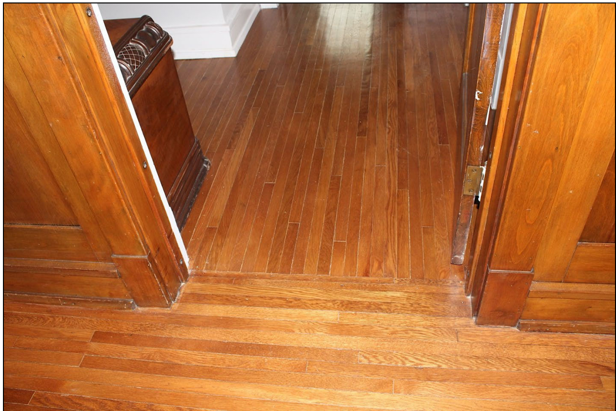
Figure 13: Threshold between hall and dining room; view facing north, 2022.
