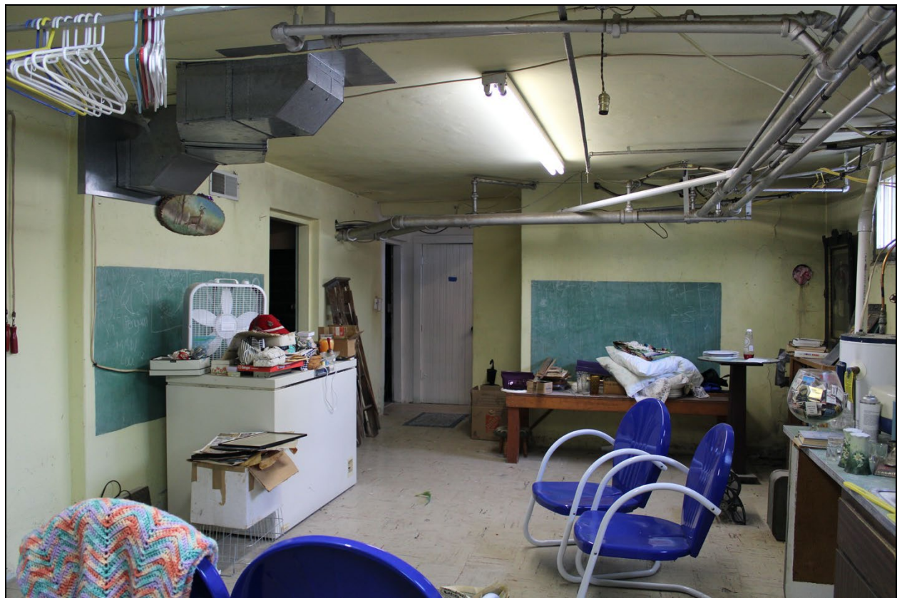
Figure 17: Basement with chalkboards; view facing north, 2022.
