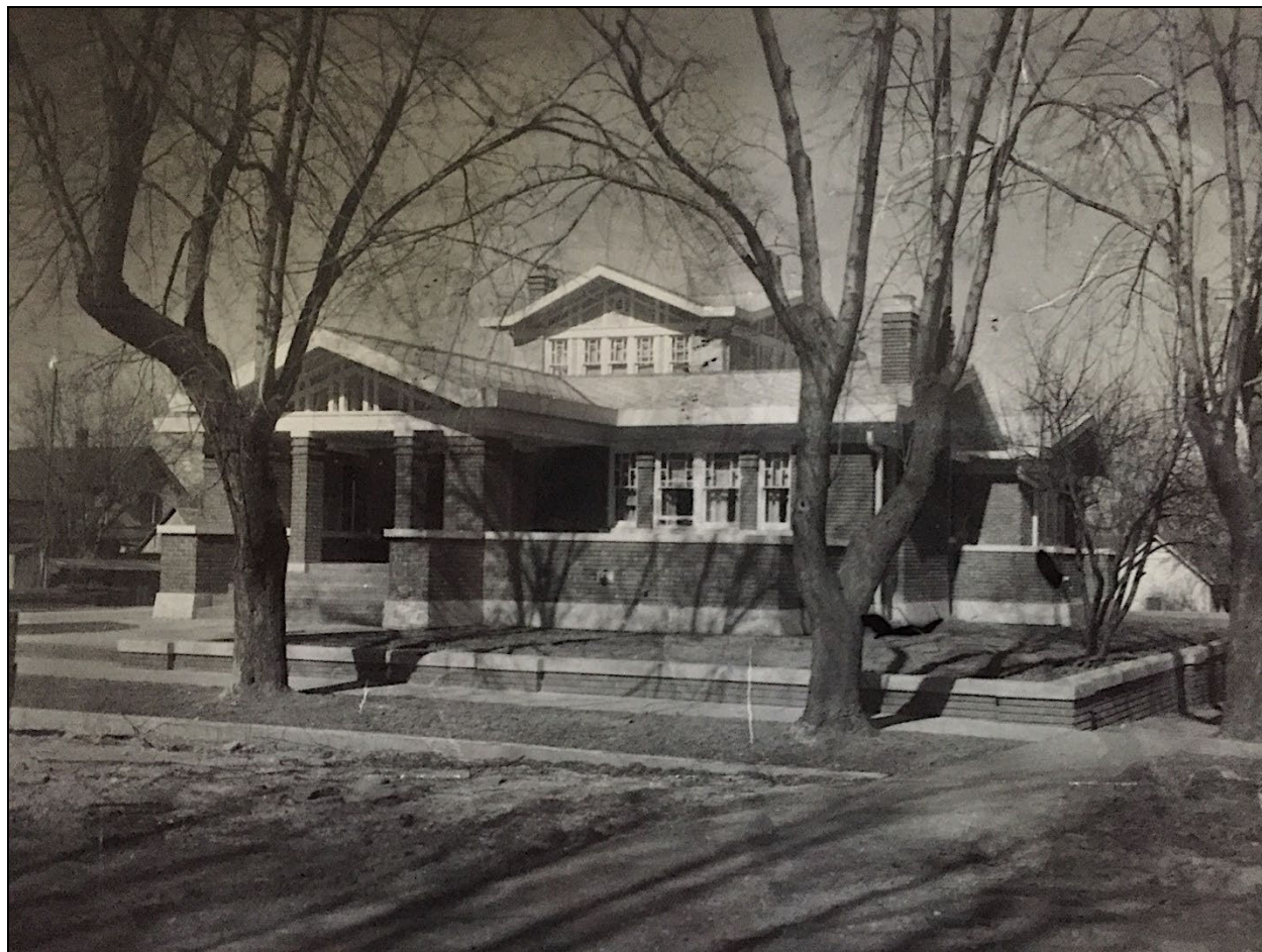
Figure 6: Historic photograph of the P. A. Switzer Residence, undated.
