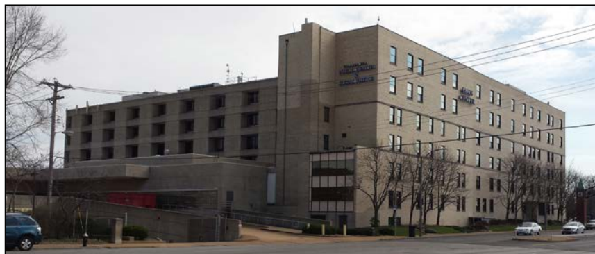
Figure 37: Incarnate Word Hospital (now St. Louis University Salus Center). The façade (right) is intact, but 1970s additions more than doubled the size of the hospital before it was taken out of use. Photo by Lynn Josse, March 2017.
