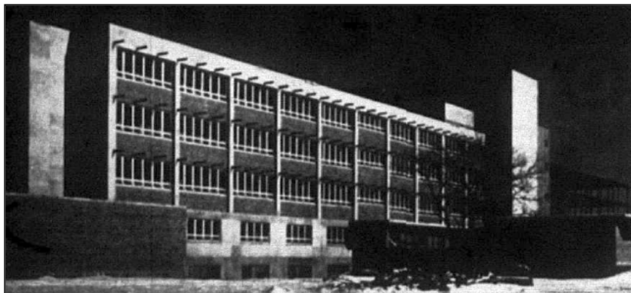
Figure 17: Rockford Memorial Hospital under construction.
