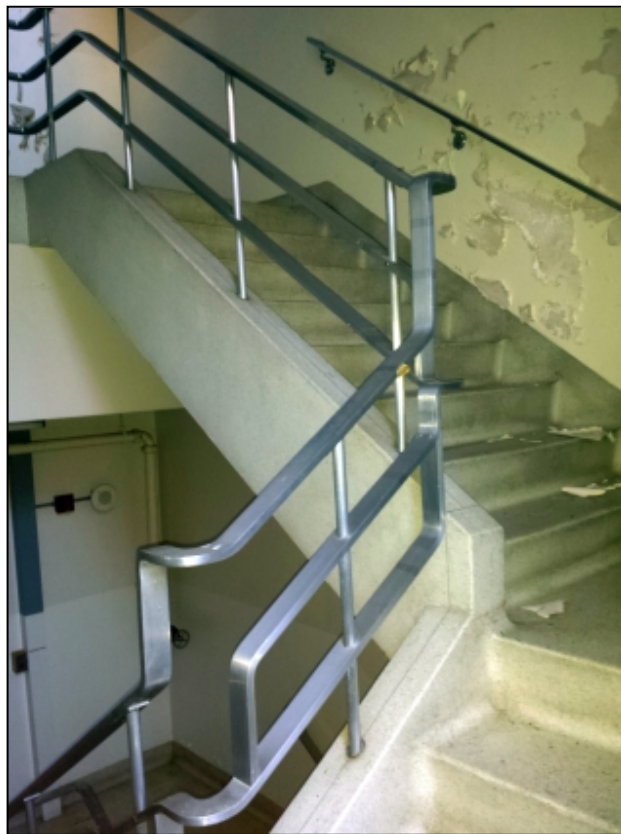
Figure 27: The Fowler Wing's main stair. Photo: Lynn Josse, March 2017.
