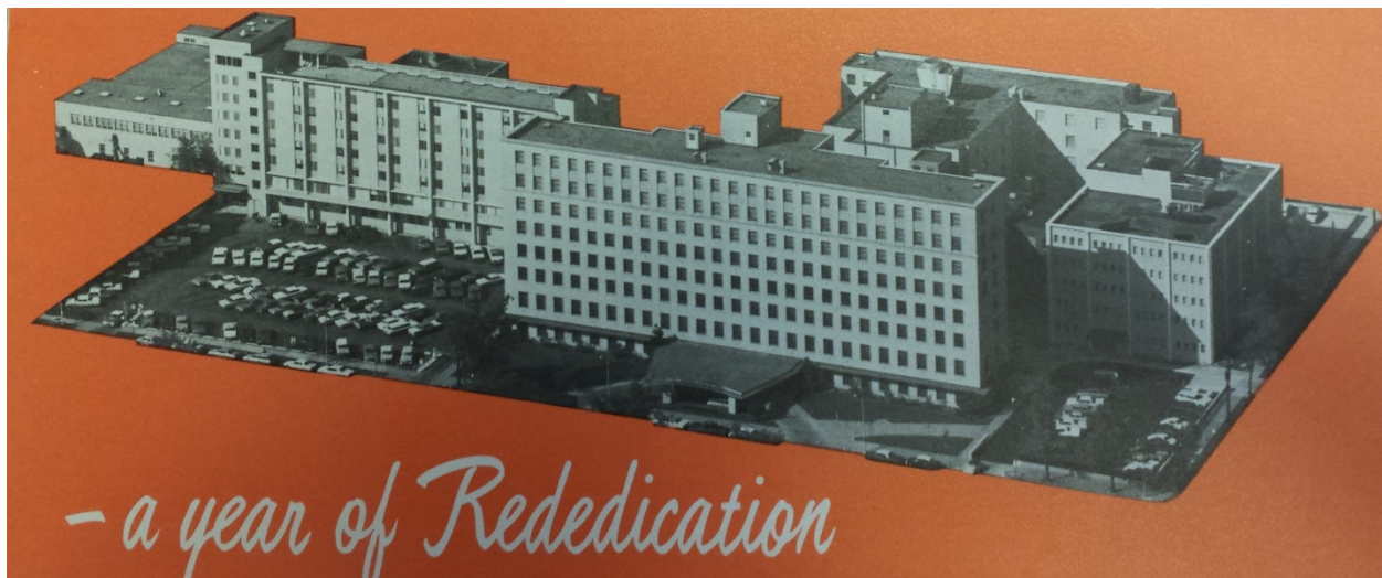
Figure 34: The cover of the 1966 Annual Report refers to "a year of Rededication" because, as the administrator explained, it was the first time in recent memory that no buildings were going up or down. The expansion envisioned in the early 1950s was finally complete. Source: 1966 Annual Report.
