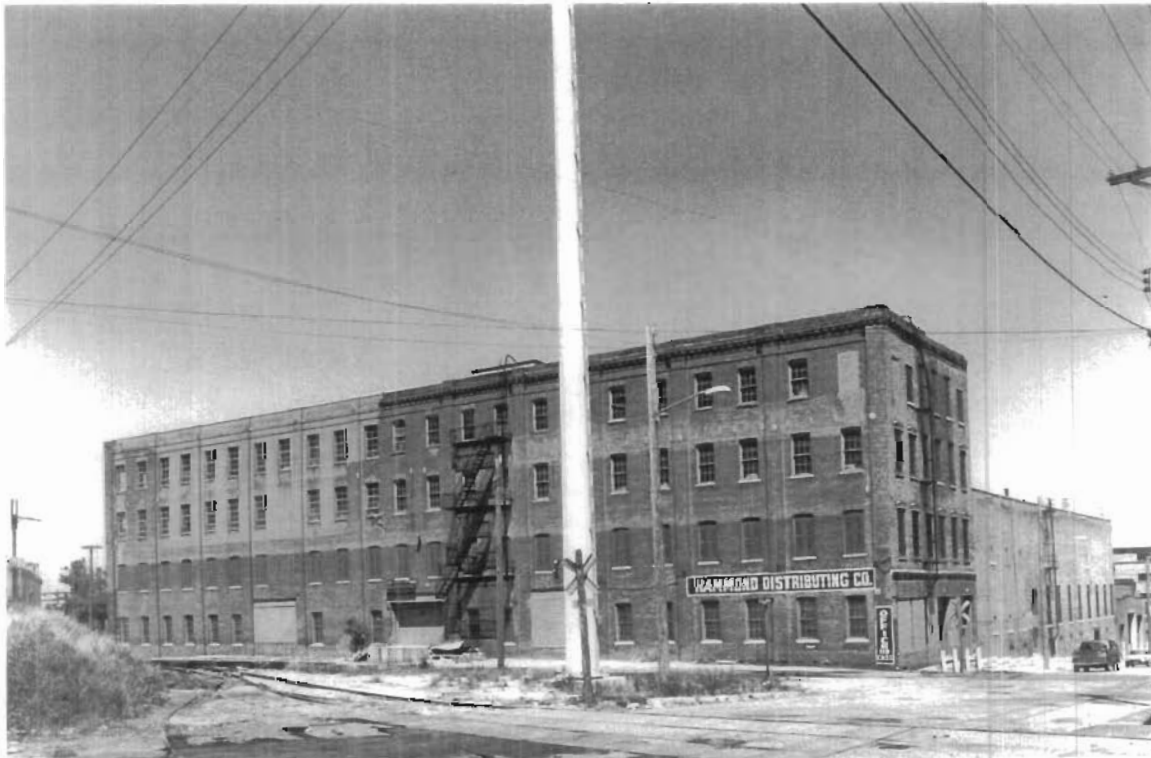
Figure 11: The St. Louis Stamping Company buildings in 1989. Note the presence of original six-over-six wooden window sash on the corner building that was later covered by corrugated plastic sheeting. (Source: Survey of the North Riverfront Industrial Area by Landmarks Association of St. Louis.)
