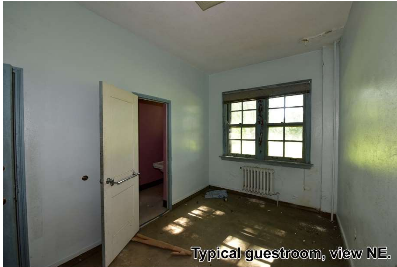
Figure 16. Typical Gethsemane Retreat House finishes. Source: Brad Finch, 2020.
