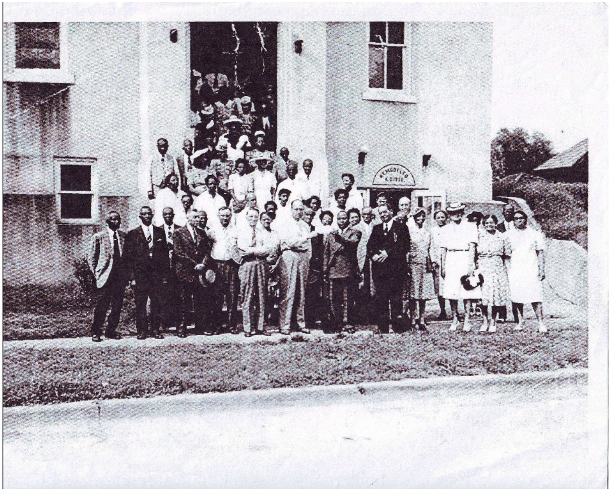
Mortgage Burning, August 5, 1945. Note the original light fixtures above basement door, and relative size and scale of fixtures flanking the arched opening. Photo Source: St. James AME Church.
