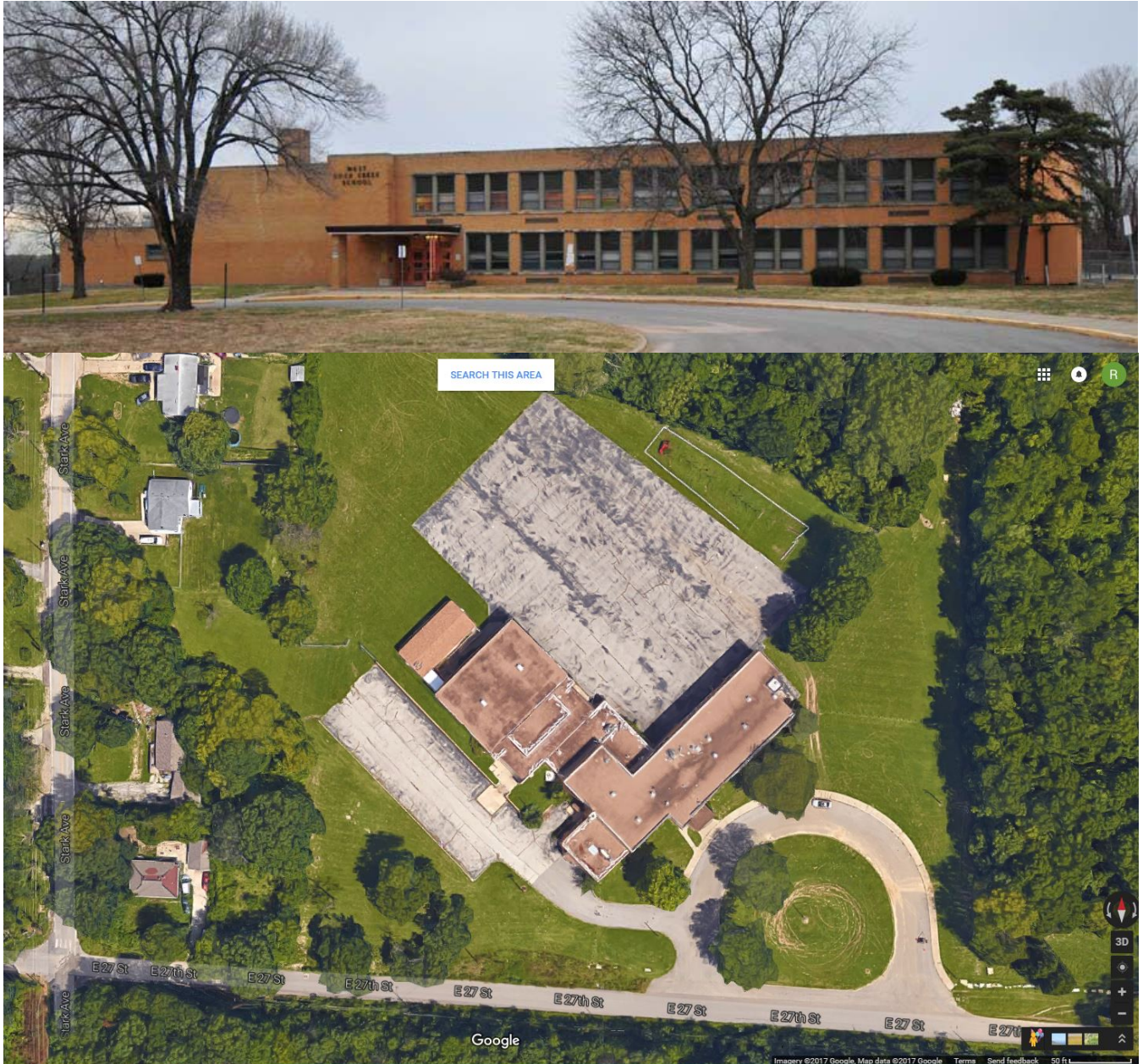
Figure 27. West Rock Creek School (8820 E. 27 th St., 1961), Kansas City Public Schools, Photo and Plan. Source: Brad Finch, 2011; Google Maps, 2017.
