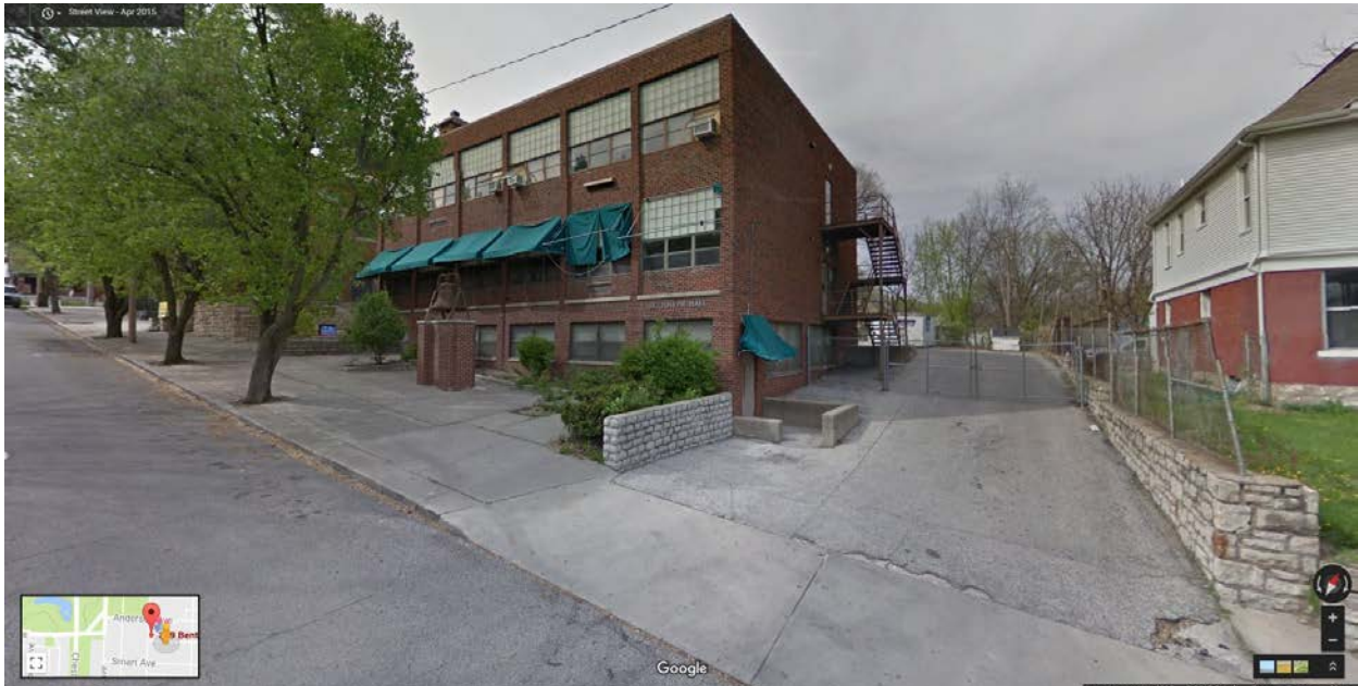
Figure 35. Assumption Parish School (309 Benton Blvd., 1954), Catholic School, Photo and Plan. Source: Google Maps, 2017.
