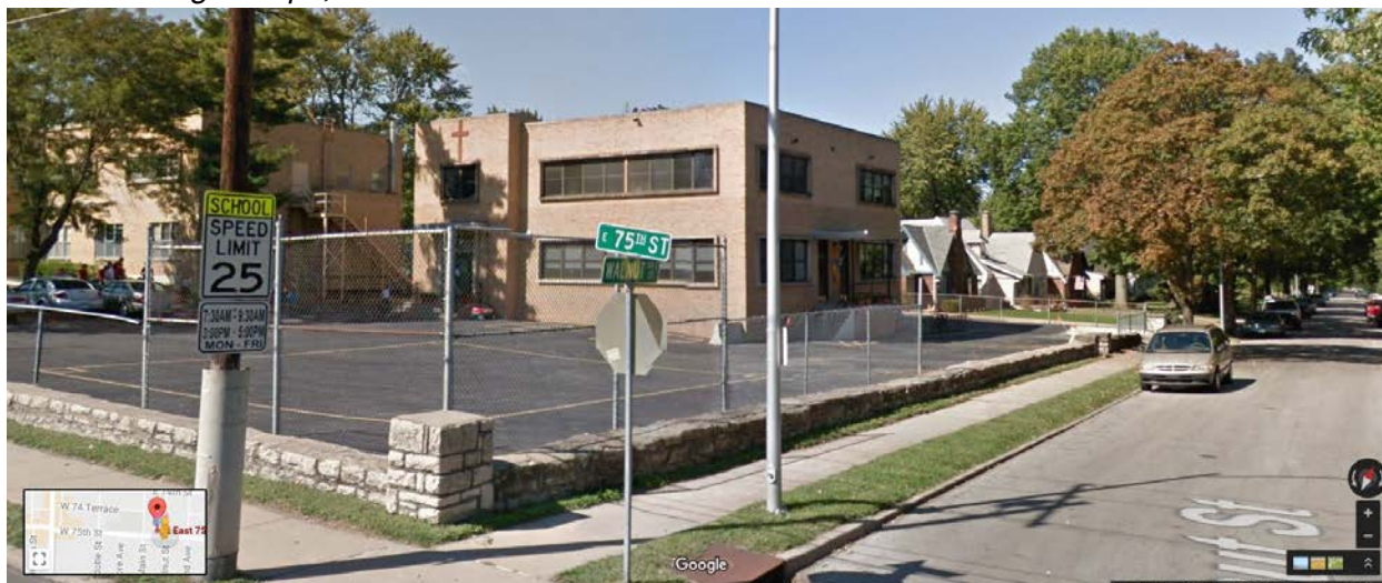
Figure 33. St. Elizabeth's Parish School (2 E. 75 th St., 1953), Catholic School, Photo and Plan. Source: Google Maps, 2017.
