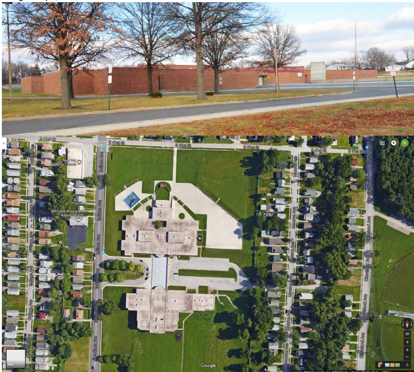
Figure 30. Weeks Elementary School and Martin Luther King, Jr. Middle School complex (4201 Indiana Ave., 1968), Kansas City Public Schools, Photo and Plan. Source: Brad Finch, 2011; Google Maps, 2017.
