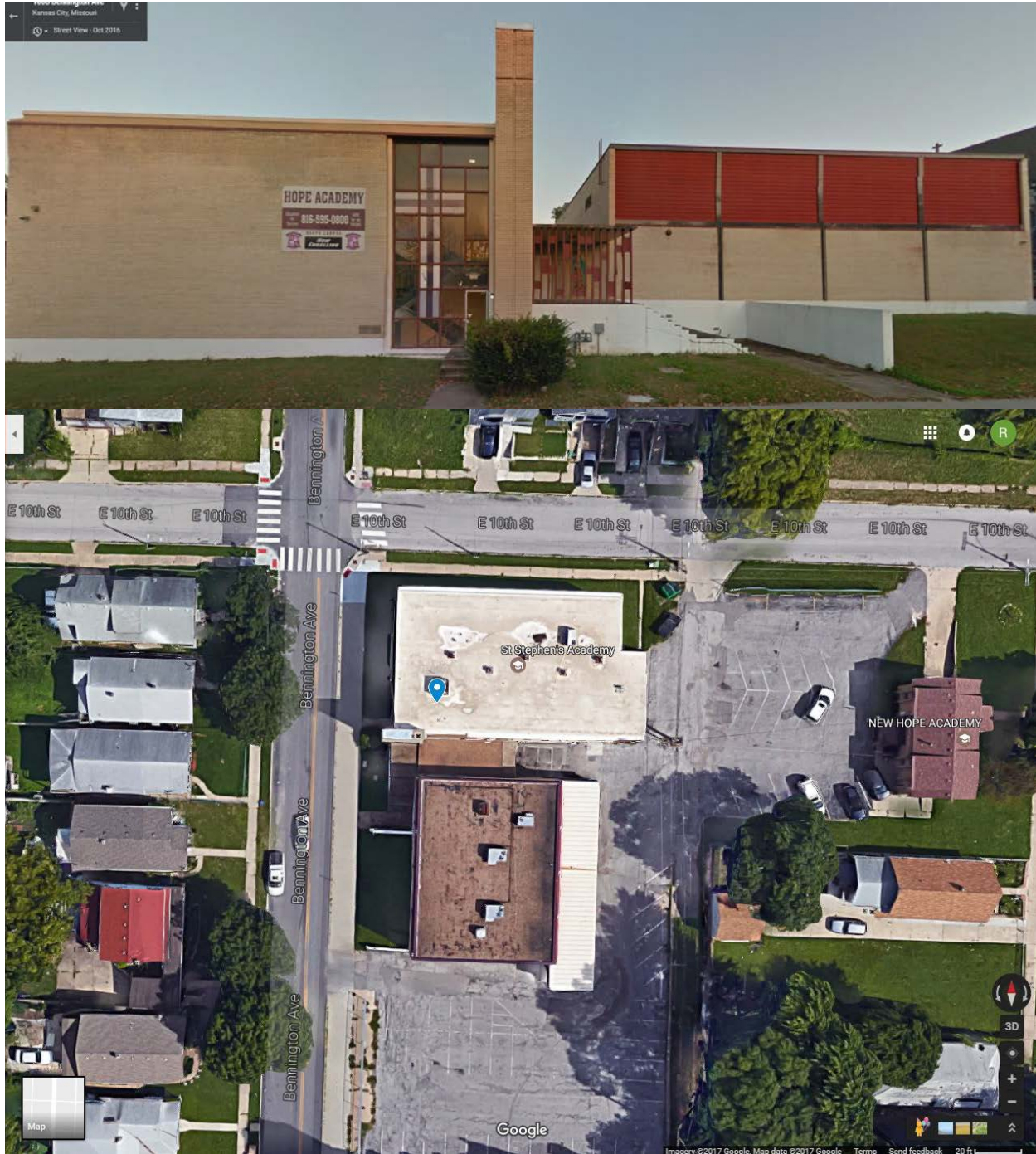
Figure 40. St. Stephen's Parish School (1025 Bennington Ave., 1959), Catholic School, Photo and Plan. Source: Google Maps, 2017.
