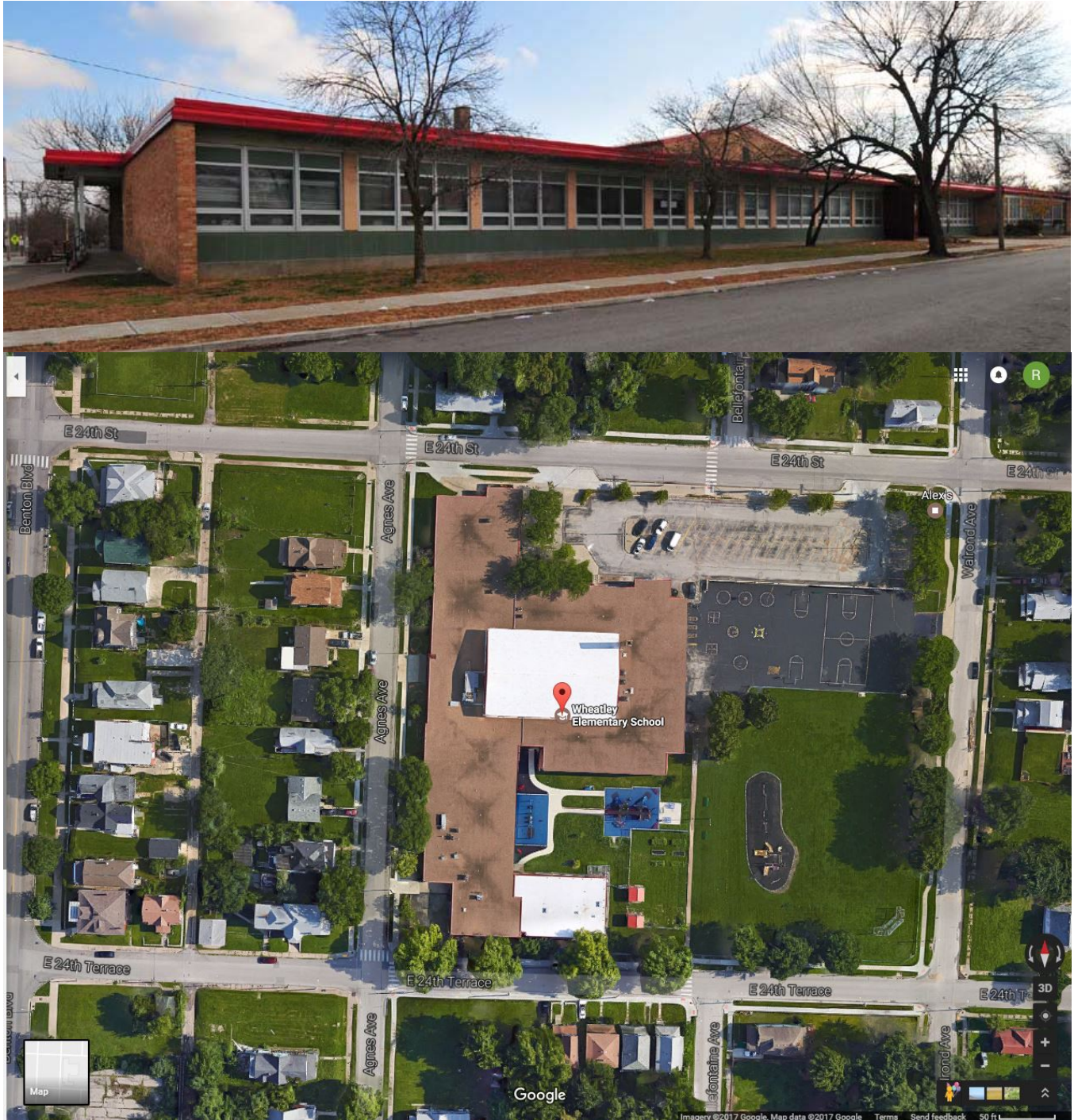
Figure 22. Wheatley School (2415 Agnes Ave., 1955), Kansas City Public Schools, Photo and Plan. Source: Brad Finch, 2011; Google Maps, 2017.
