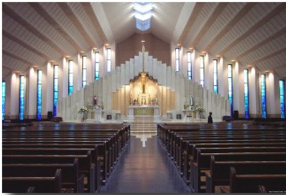
Figure 26. Church of Christ the King, Cork, Ireland. View toward the altar (top); exterior (bottom left); detail of entry (bottom right). Sources: Church of Christ the King website (top, bot left); Felicity Rich, photographer in Michael, The Architecture of Barry Byrne , 96.
