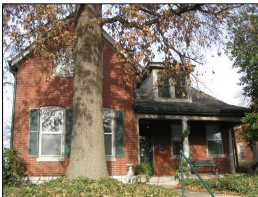
626 Clark Street. Right side-gabled wing built circa 1864, gable-front wing and Colonial Revival gallery added circa 1923
