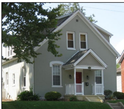
1009 North Fifth Street, 1890. This house is the earliest example of a Gable Front cottage in the survey area.
