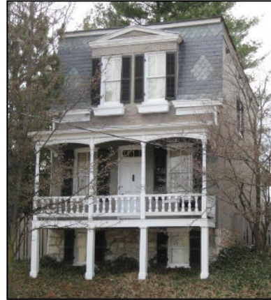
607 North Fifth Street, circa 1870. This house has a front mansard roof and a raised basement.
