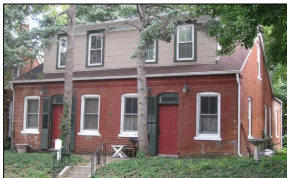
720 North Benton Avenue. The north (left) half of this house was built in the early 1870s and the south (right) half was added later to create a duplex.
