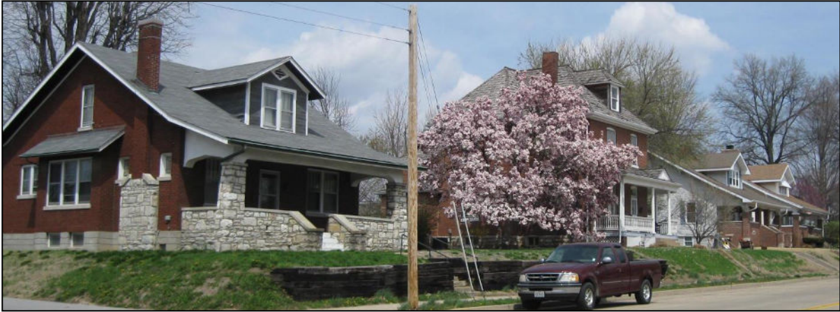
The houses at 1101-1125 North Fifth Street include a Craftsman Bungalow, a 2 ½-story Queen Anne Free Classic style house, and two vernacular Bungalows.
