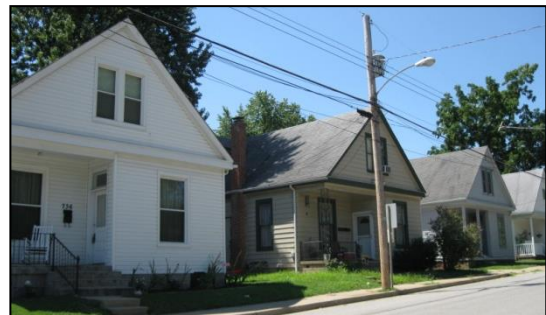
A row of four Gable Front cottages with recessed corner porches is in the 700 block of North Kingshighway.
