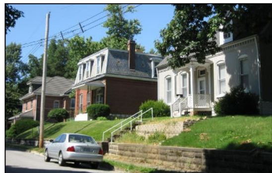
631-705 North Benton Avenue. Many lots are elevated above the street and have retaining walls.
