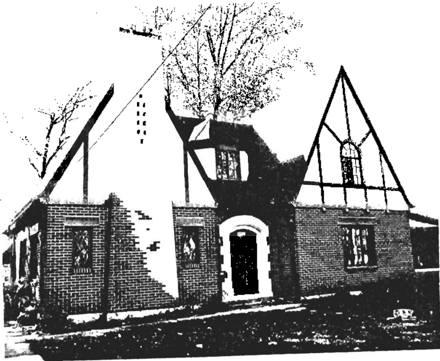
English Cottage revival house style. 1230 East Walnut Street. Built 1932-1933
