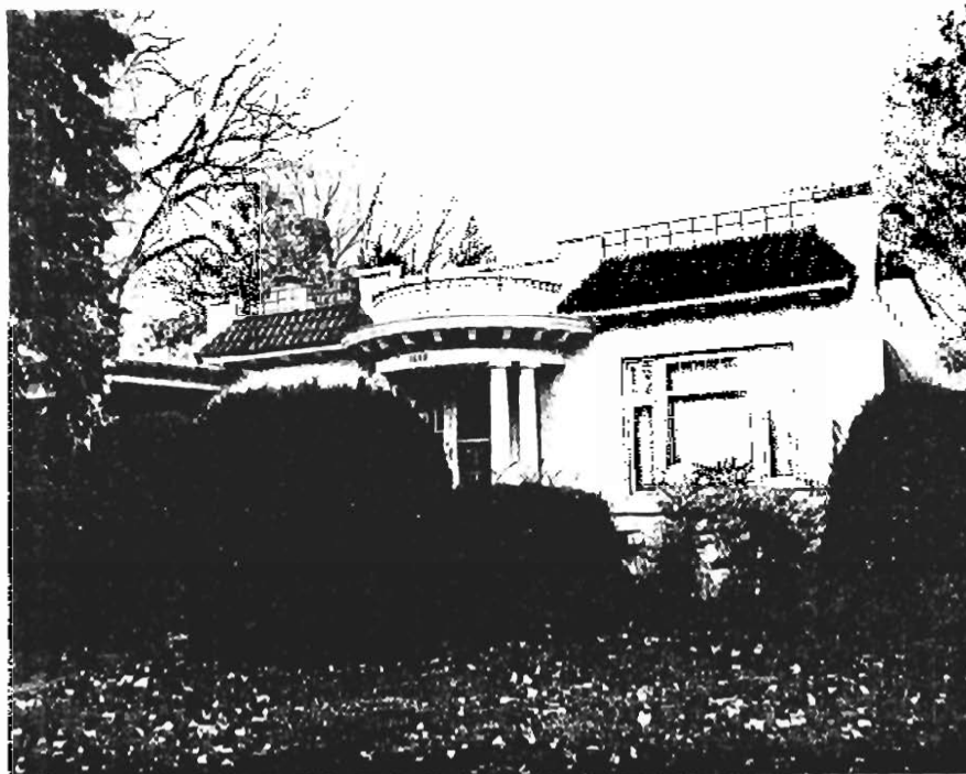
American Colonial revival house style. 1300 East Walnut Street. Built 1921-1922
