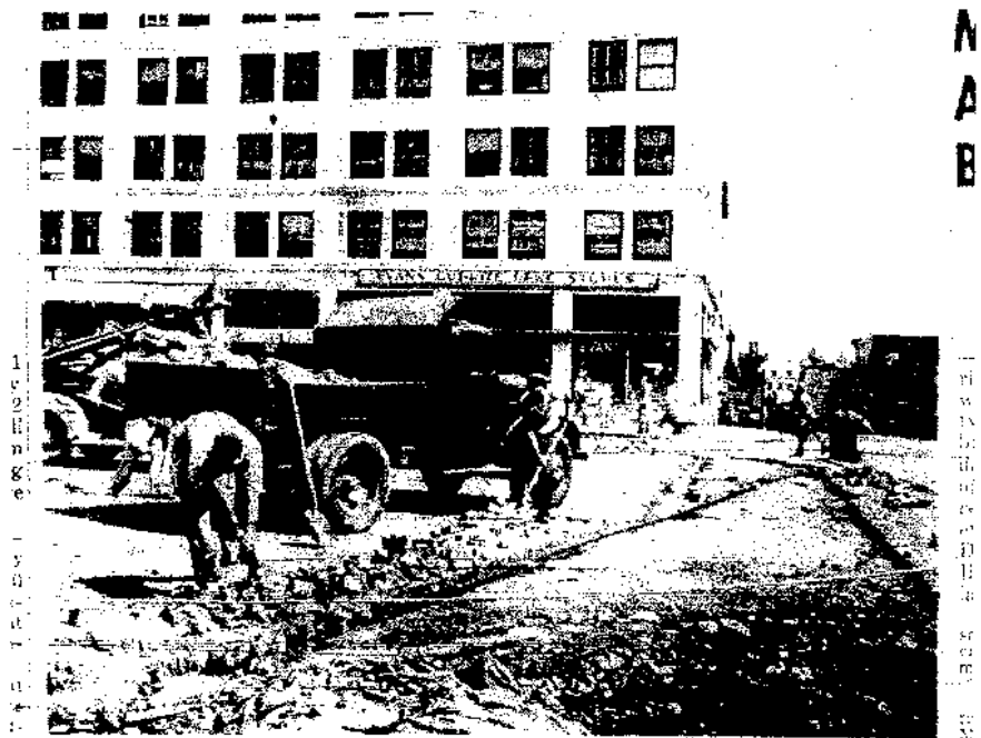
WALKWAYS FOR THE SQUARE —The excavation which you see in this picture marks the location of the sidewalk which will use in crossing the northwest section of Springfield's new Public Square. The eight-foot walkways will border each of the Square's new parking areas, and also will mark the boundaries of the new traffic signals to guide both pedestrian and vehicular traffic. This northwest parking area will be completed this week, and workmen then will proceed to the northeast section. Meanwhile, with completion of underground work on the south side of the Square, that section will be opened to traffic on Thursday morning. When the northern parking areas are finished, work will begin on the two southern sections, which then of course must be barricaded again.
