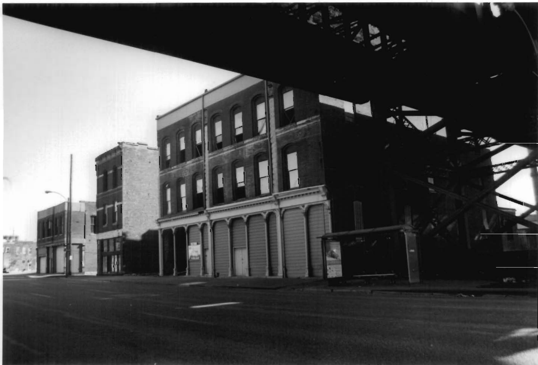
South Fourth Street Commercial District St. Louis (Independent City), Mo. Photo # 1
