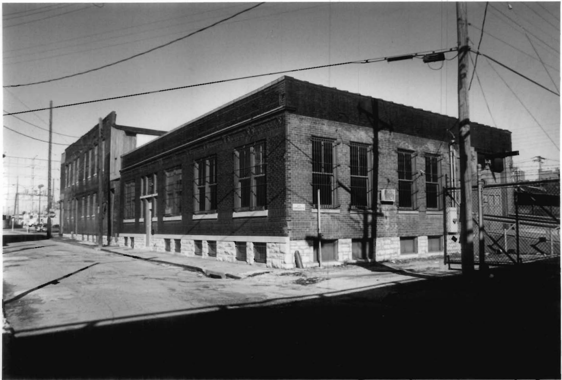
South Fourth Street Commercial District St. Louis (Independent City), MO. Photo # 3
