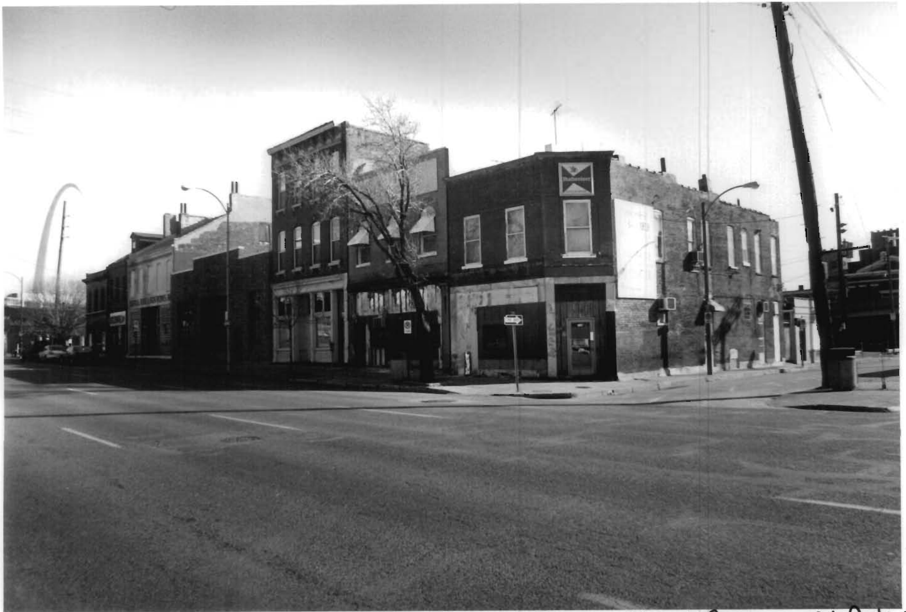
South Fourth Street Commercial District St. Louis (Independent City), Mo. Photo # 4
