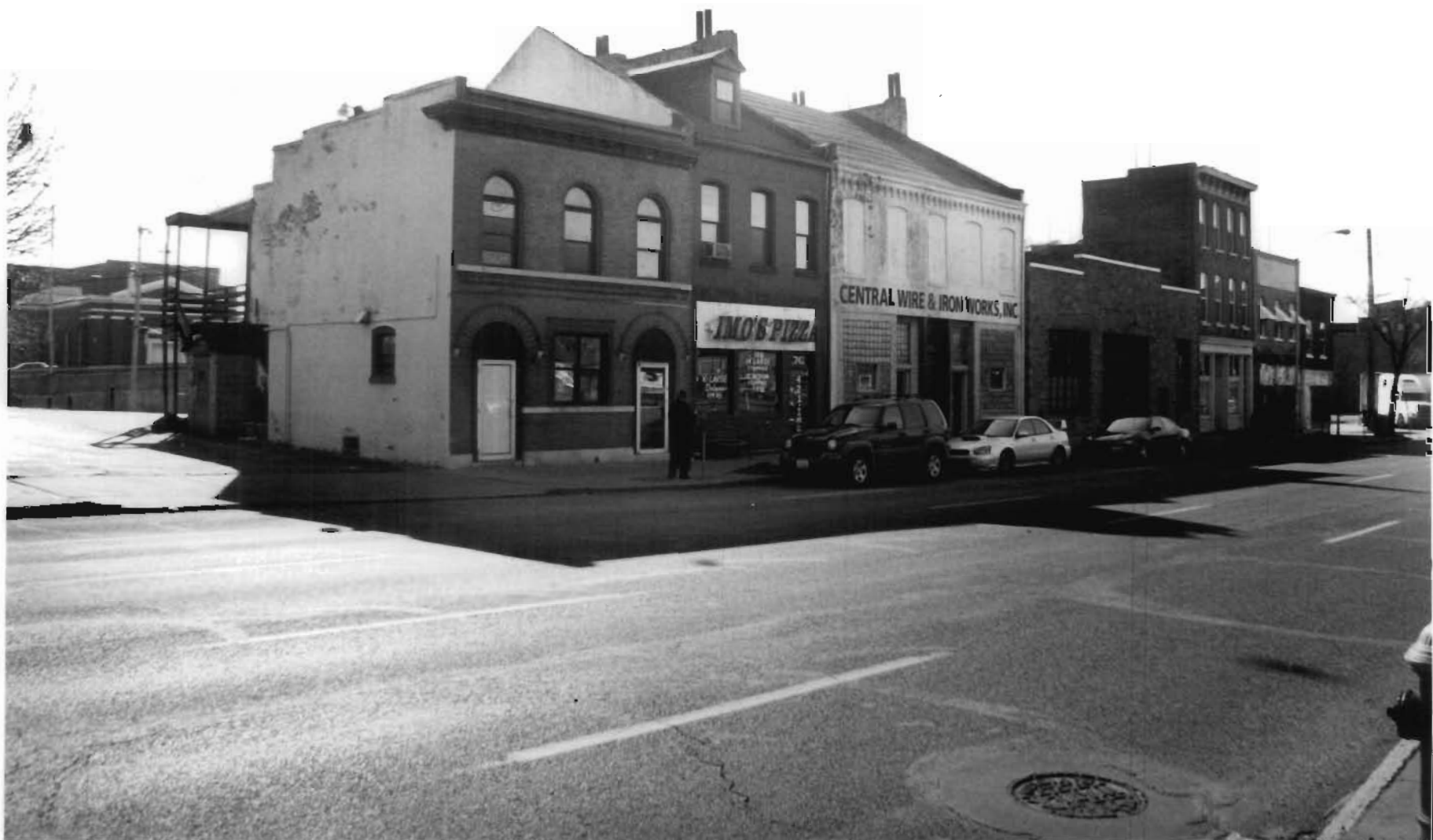
South Fourth Street Commercial District St. Louis (Independent City) Mo. Photo # 5
