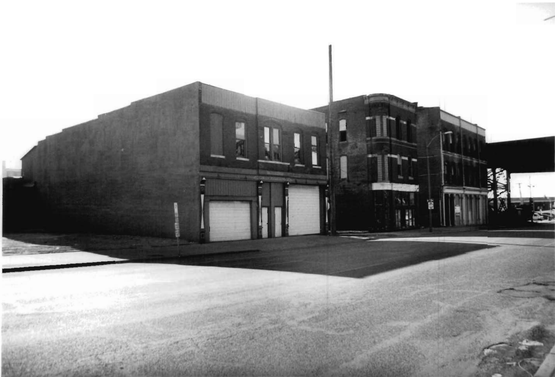
South Fourth Street Commercial District St. Louis (Independent City), MO. Photo # 2
