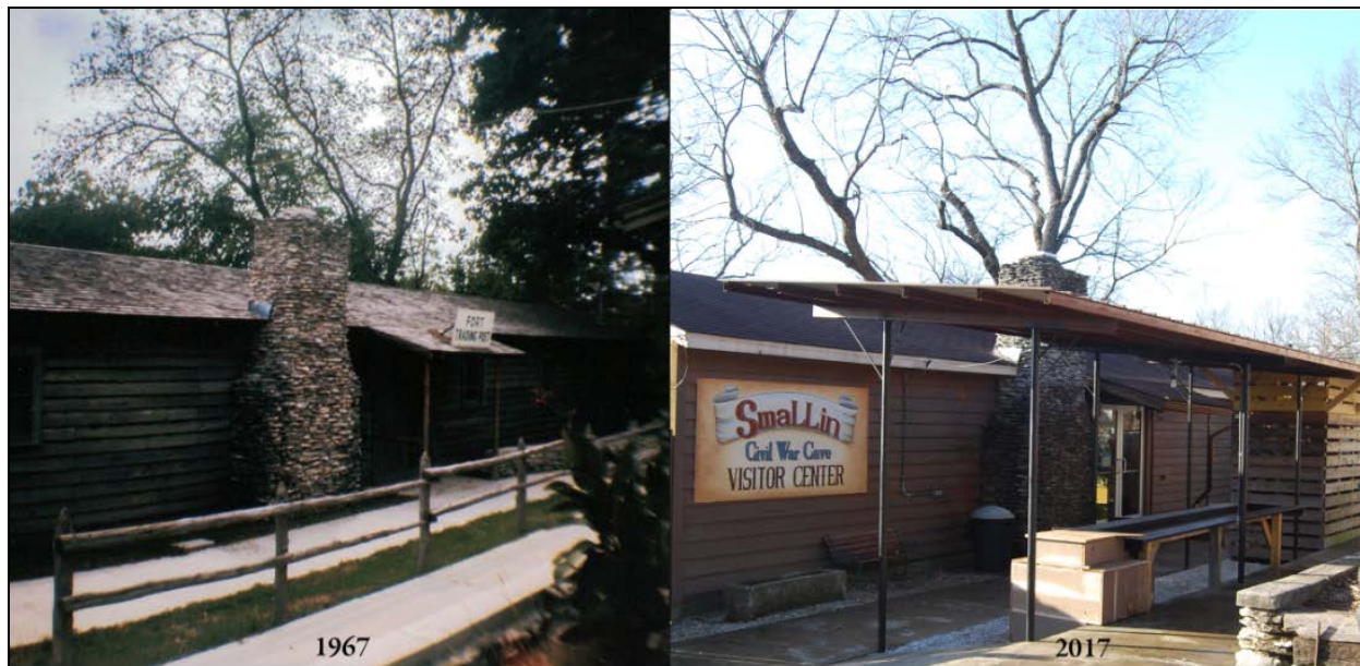
Figure 23: The Visitor's Center Then and Now, North Elevation. The north elevation of the Visitor's Center is pictured in 1967 (left) and today (right). The activity center on the left side is freestanding structure. Image provided by Kevin Bright.
