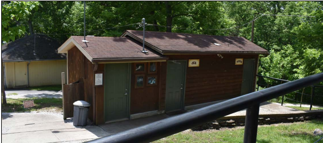
Figure 26: Restrooms (c. 1960), Contributing Building. Image taken by Michelle Diedriech, Spring 2017.
