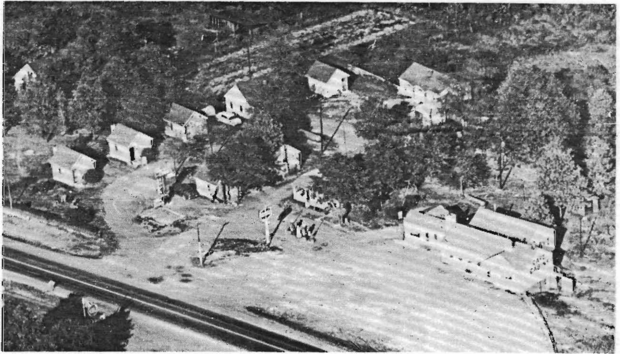
ROCK HAVEN COURT--HWY. 66-1½ MI. WEST OF ST. JAMES. MISSOURI Cabins---Good Food---Service Station
