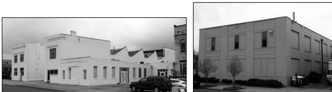
Figure 5: Left: 4011-4015 Forest Park Ave. The residential building at 4007 Forest Park is just visible at the right. The sawtooth roof is part of the A. Gilbert & Sons Foundry at 4015 Forest Park Ave. Right: Built as part of the Johnson, Stephens & Shinkle Shoe Company complex, the building at 4251 Forest Park (1925) had large windows but no overhead day lighting.
