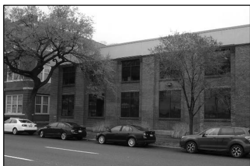
Figure 7: The Haynes-Langenberg factory (1907, 4041 Forest Park), left, can be considered Commercial Style because of its brick-clad grid allowing for wide window openings. It is not known what the original cornice looked like. See also 4210 Forest Park Avenue in Figure 6.
