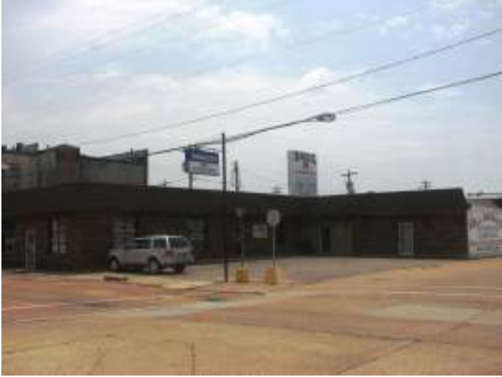
Façade (north and west elevation, showing off street parking)
