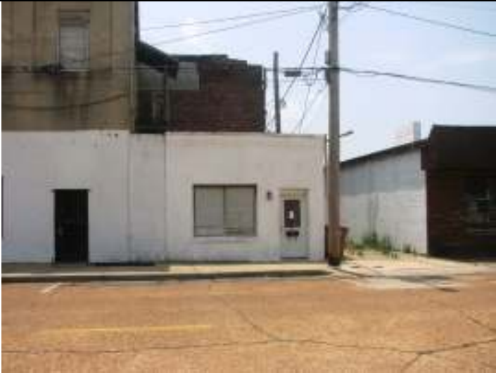
Façade (north) – showing building adjoined to 201 S. Broadway
