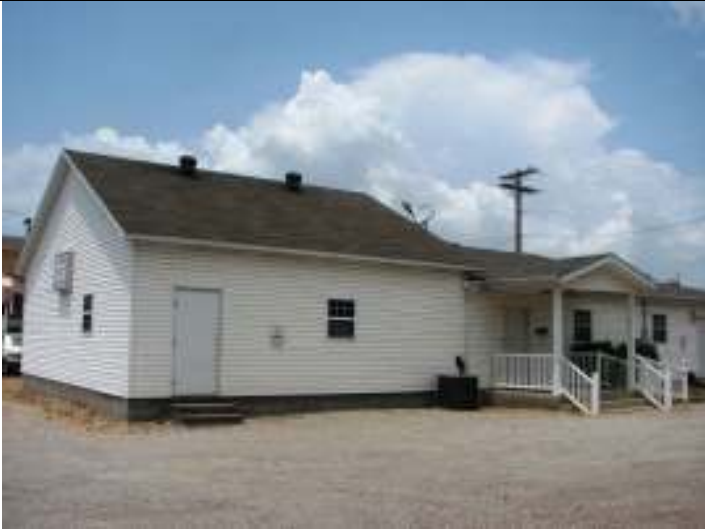
Façade (east) and south elevation
