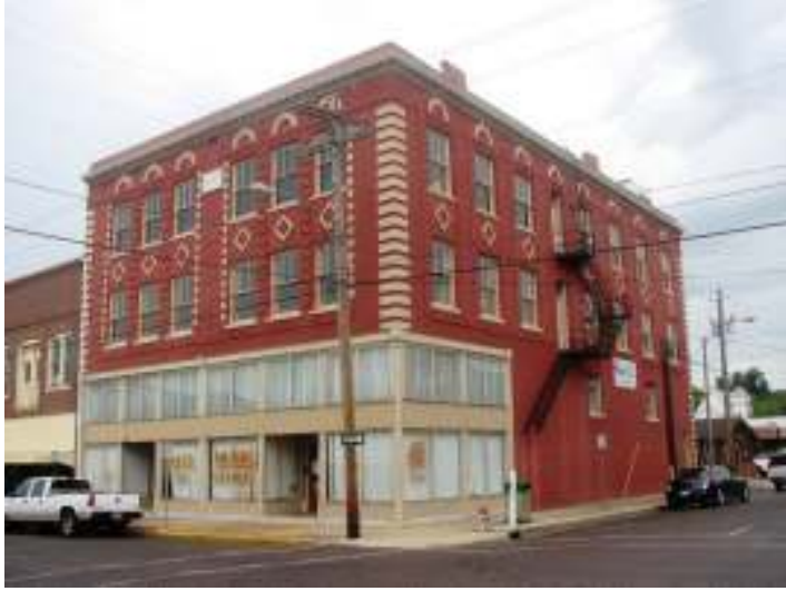
Façade (south) and east elevation
