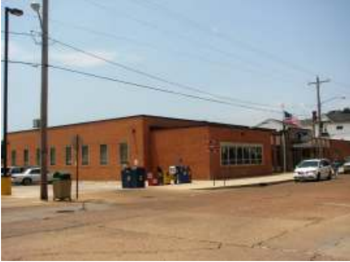
Façade (north) and east elevation
