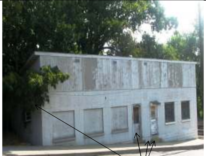
Façade, showing missing step, crack in foundation, deteriorated doors and overgrown vegetation
