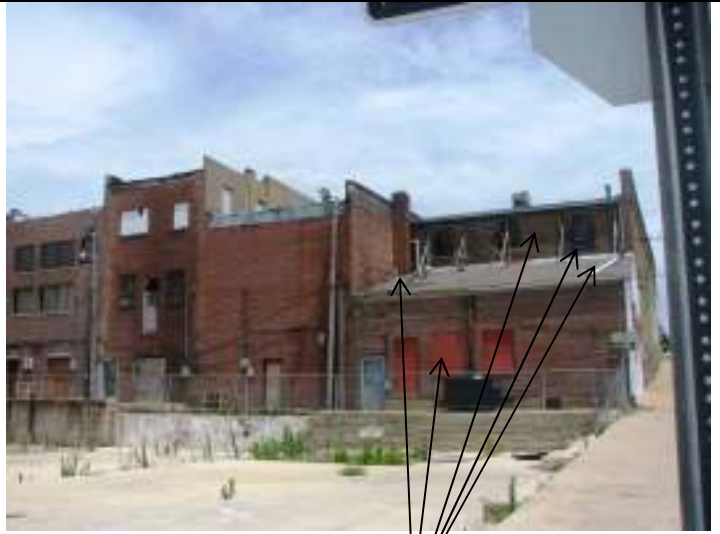
West elevation, showing boarded up windows, gutters but no downspouts, and mortar issues
