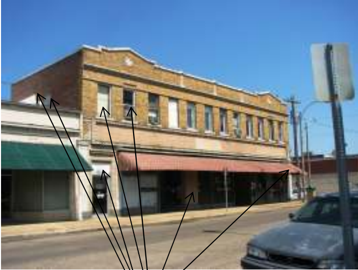
Façade (east) and south elevation showing bent awning, boarded up windows, missing windows
