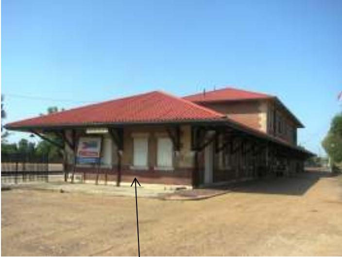
North elevation, showing boarded up windows
