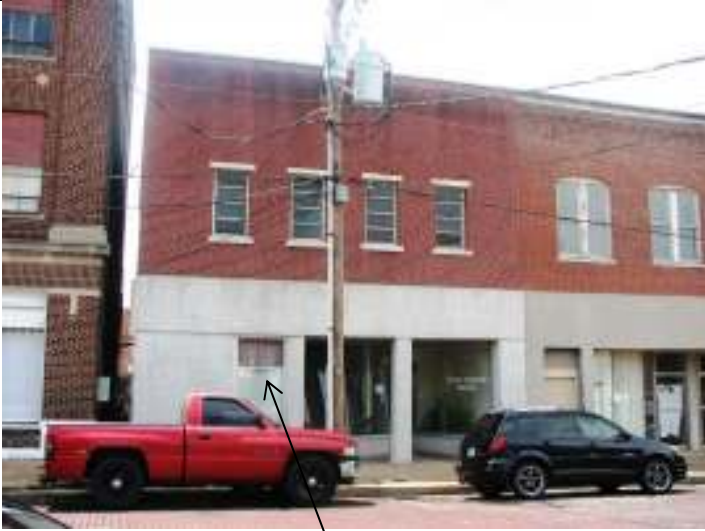
Façade (east), showing infilled window opening
