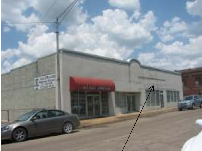
Façade (east), showing missing awning cover
