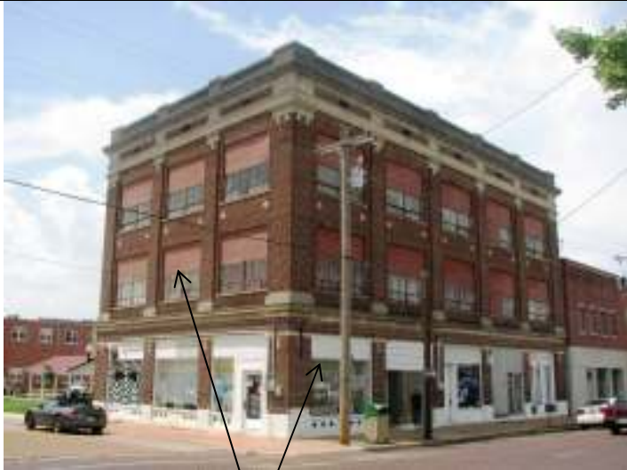
Façade (east) and south elevation, showing boarded up windows
