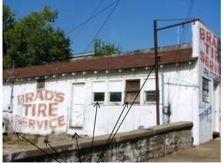
East elevation, showing boarded window, missing entrance step, loose siding and missing shingles
