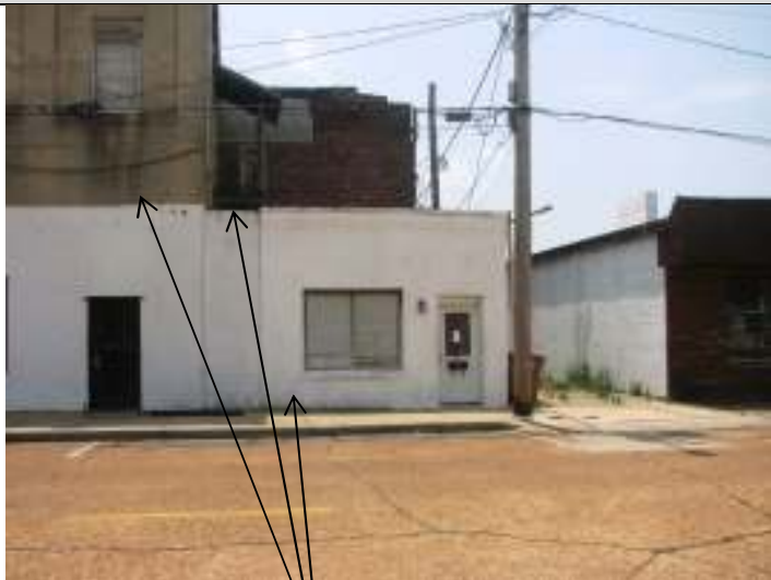
North and west elevation, showing weathered stucco and porch; attached building with address of 408 Poplar St.
