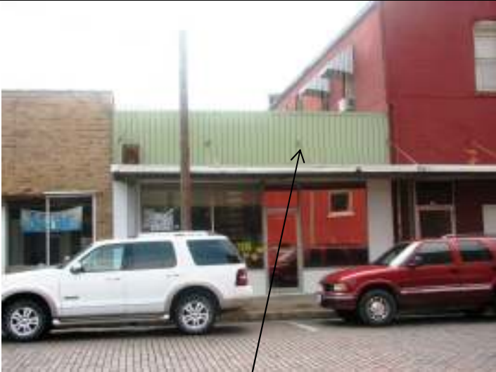
Façade (west), showing weathered supports
