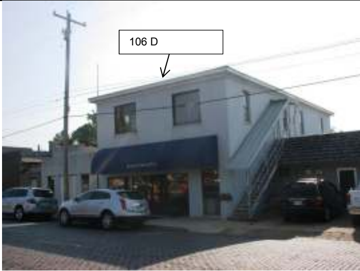
Façade (west) and south elevation
