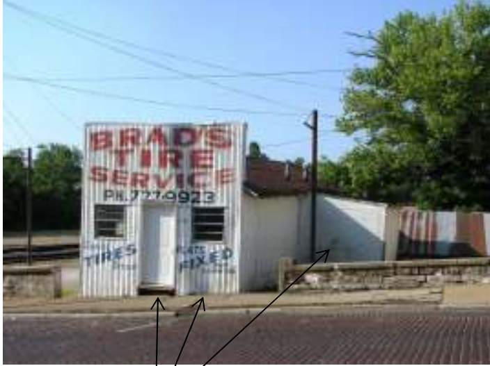
Façade (north) and west elevation, showing missing entrance step, worn siding, and metal slip cover
