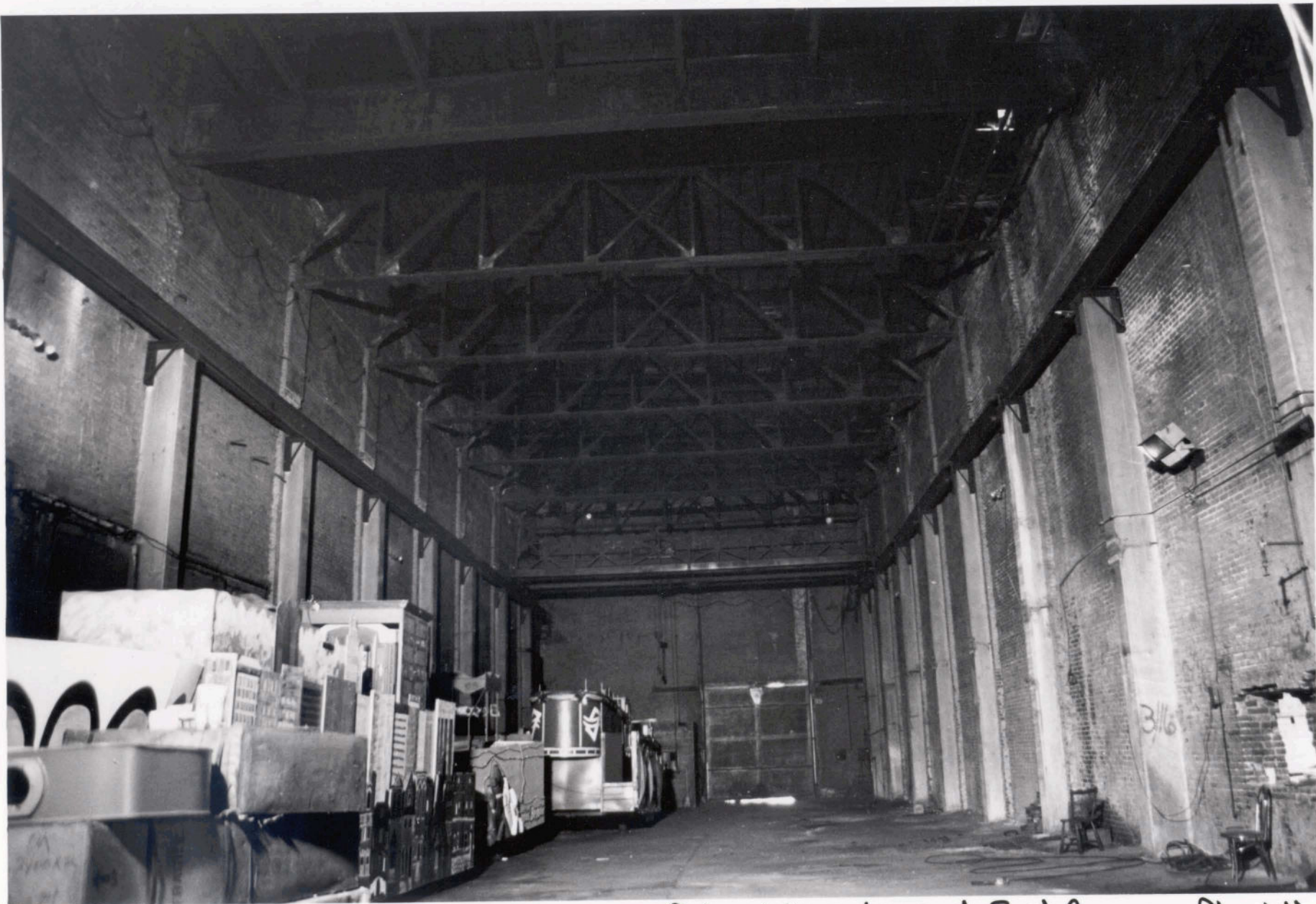
Polar Wave Ice and Fuel Company Plant No. 6 St. Louis (Independent City) Mo. Photo # 11
