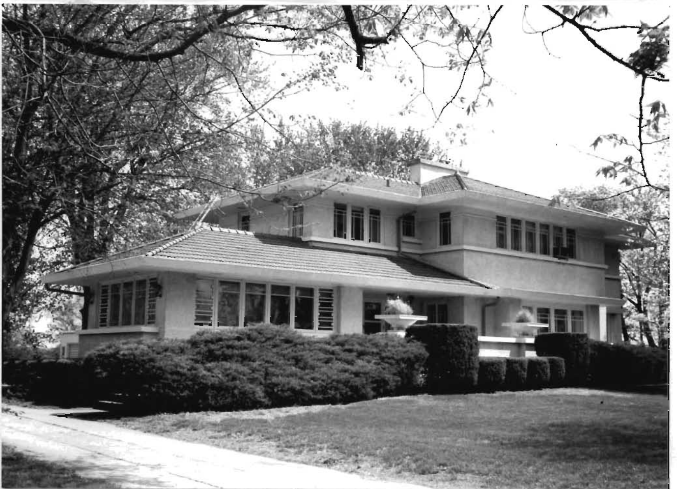
Buildings on South Main south of proposed South Palmyra Historic District
