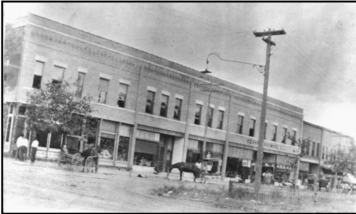
Figure 7. West side square (101-111 South Second Street) viewing WNW with new unified façade constructed after fire c. 1909-1910 (113 & 115/117 North Second Street at far right) (photo c. 1910).
