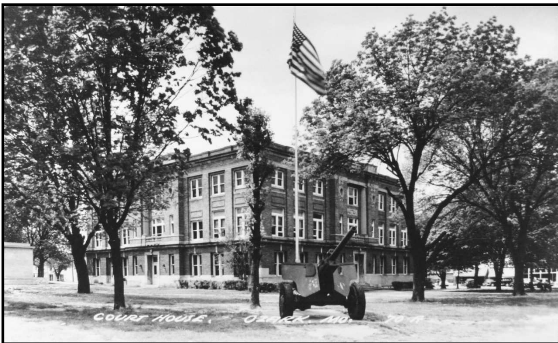
Figure 24. Courthouse viewing SW, prior to door & window replacements (photo c. 1960s).
