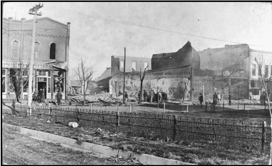
Figure 5. West side square viewing WNW, c. 1909-1910 fire destroyed 105 & 107, And gutted 109/111 Second Street (photo c. 1910).
