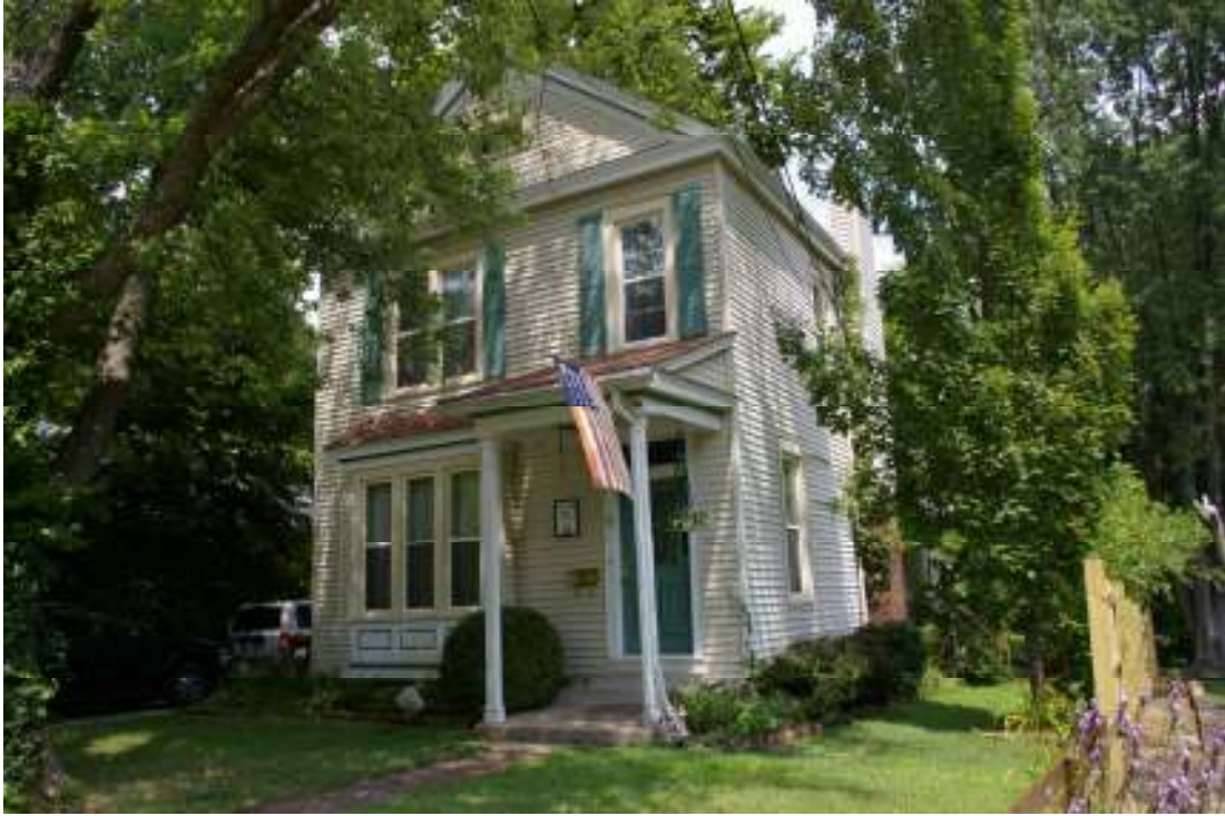
Figure 8. 18 Georgia Avenue (George S. Case Tract). The dwelling is believed to have been constructed for Peter Camden Case, son of George S. Case, c. 1887. View is facing southwest.
