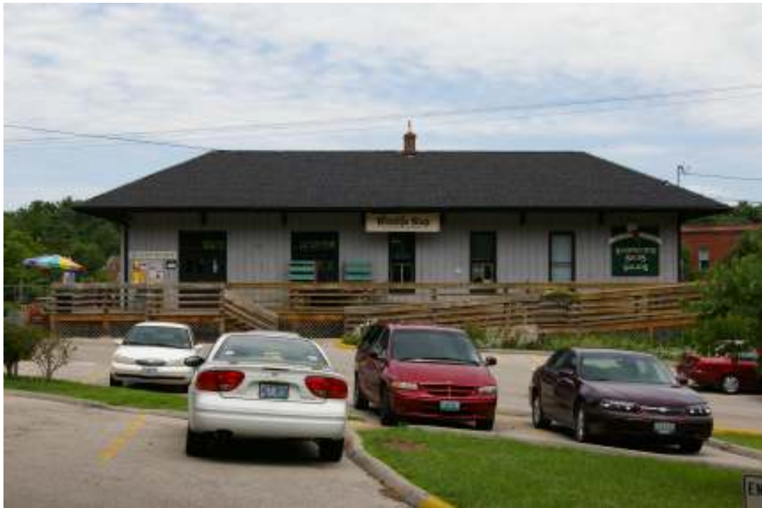
Figure 6. 1 Carson Road – formerly the Wabash train depot. This property lies within Old Ferguson West's earliest subdivision, Ashbrook Place. View is facing north.
