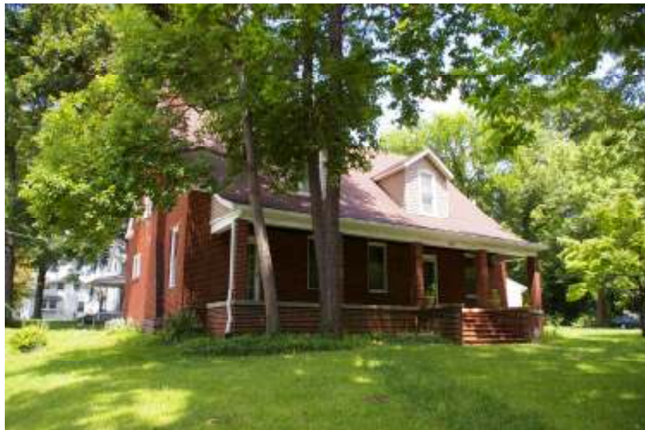
Figure 3. 125 Tiffin Avenue. The dwelling is believed to have originally served as Ferguson's first Methodist Church. It was remodeled as a dwelling in 1912, and exterior brick was added in 1927. View is facing northeast.
