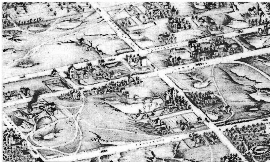
Figure 8: Sinkholes Near Jefferson and Cherokee Streets, 1875 32
