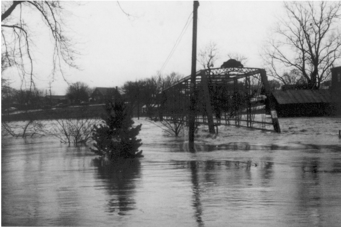
Old Appleton Bridge (During the flood of 1982) Cape Girardeau County, MO Photographer: Mary Jane Buchheit Date: December 3, 1982 Negative: Mary Jane Buchheit, Old Appleton, MO Standing in Cape Girardeau County looking north Photo 2 of 6
