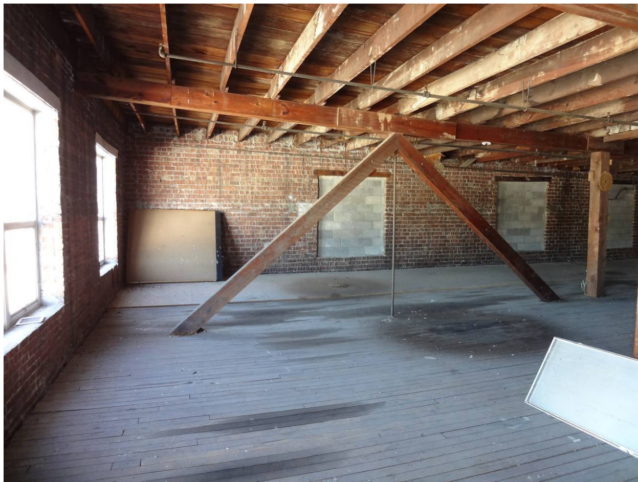
Photo 15. South third floor, looking south.
