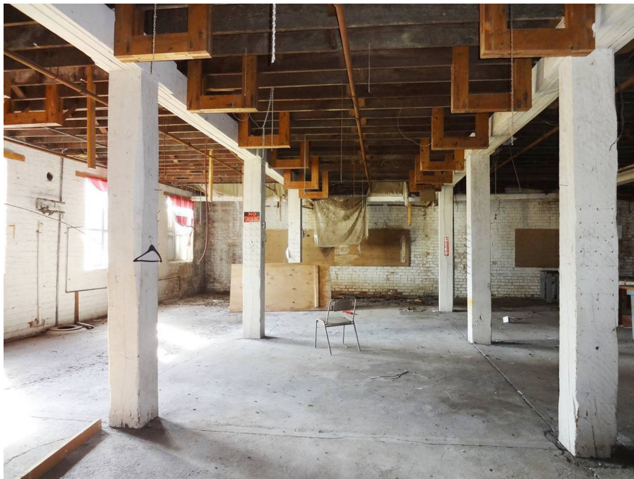
Photo 10. South ground floor interior, looking west.
