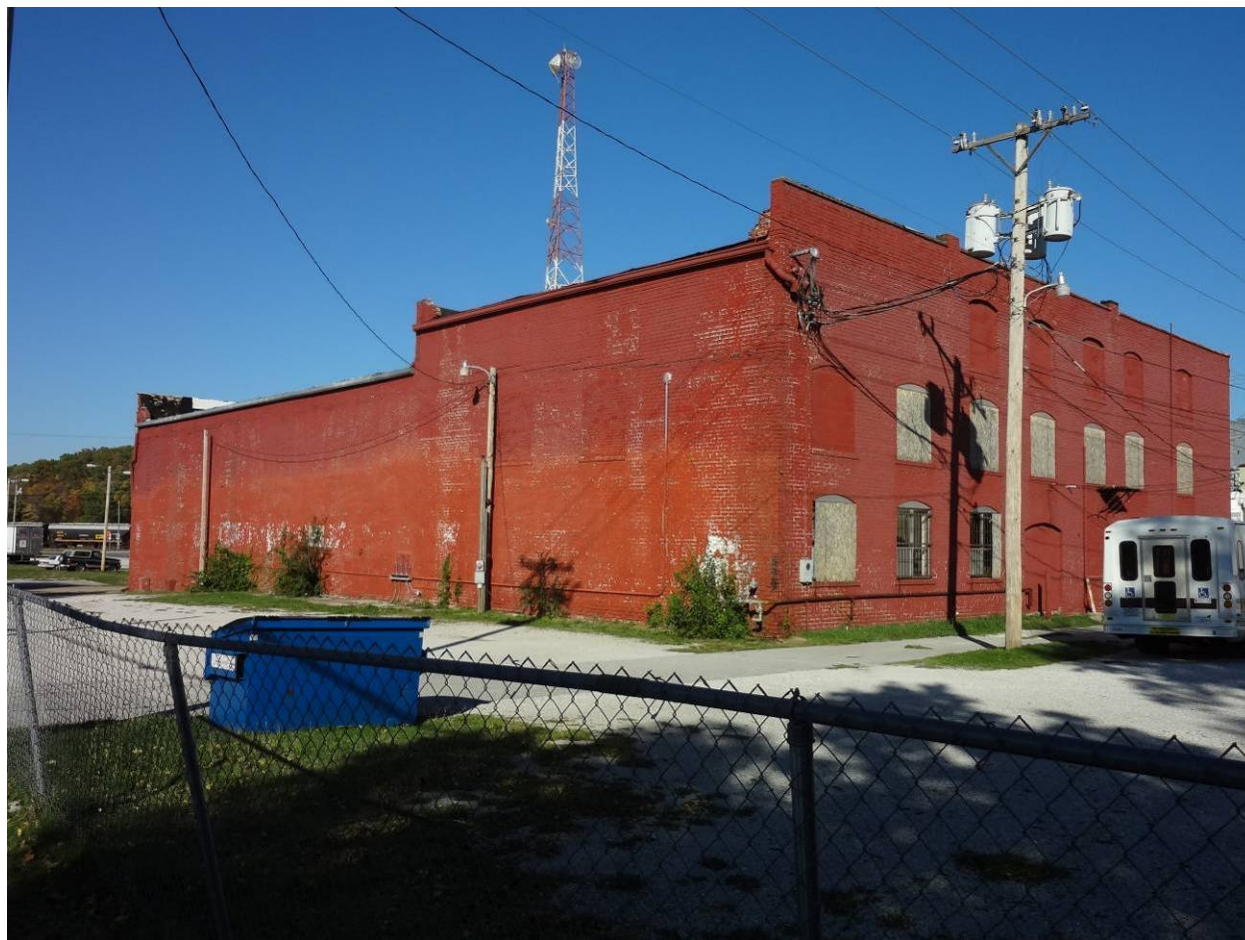
Photo 9. Southwest corner and south wall.
