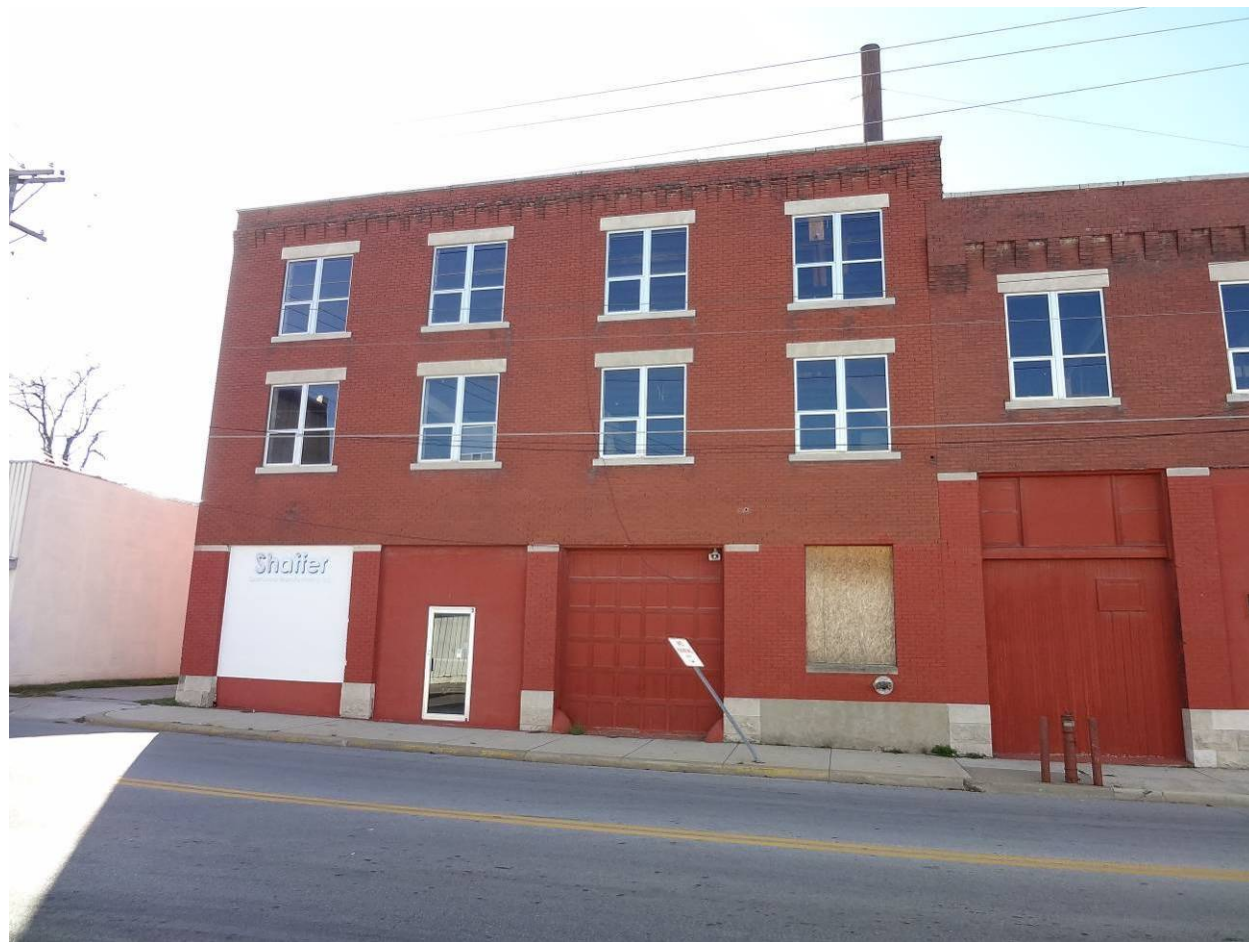
Photo 2. South end of façade. (East wall)
