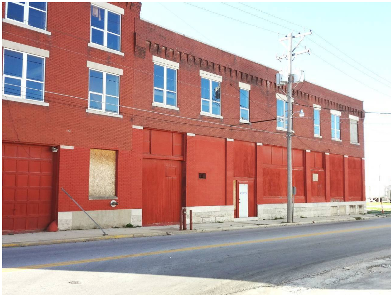
Photo 3. North end of façade.
