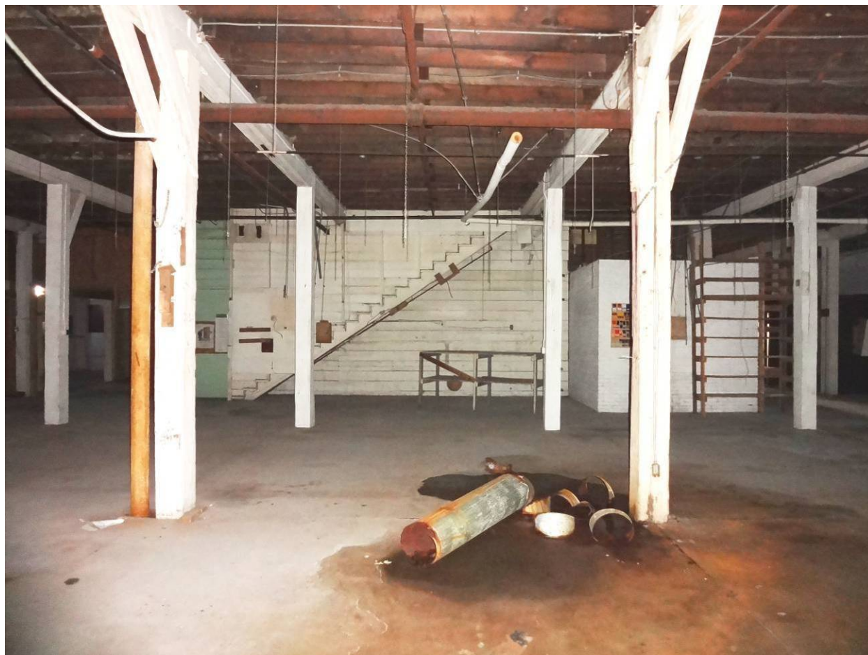
Photo 11. North ground floor, looking east.
