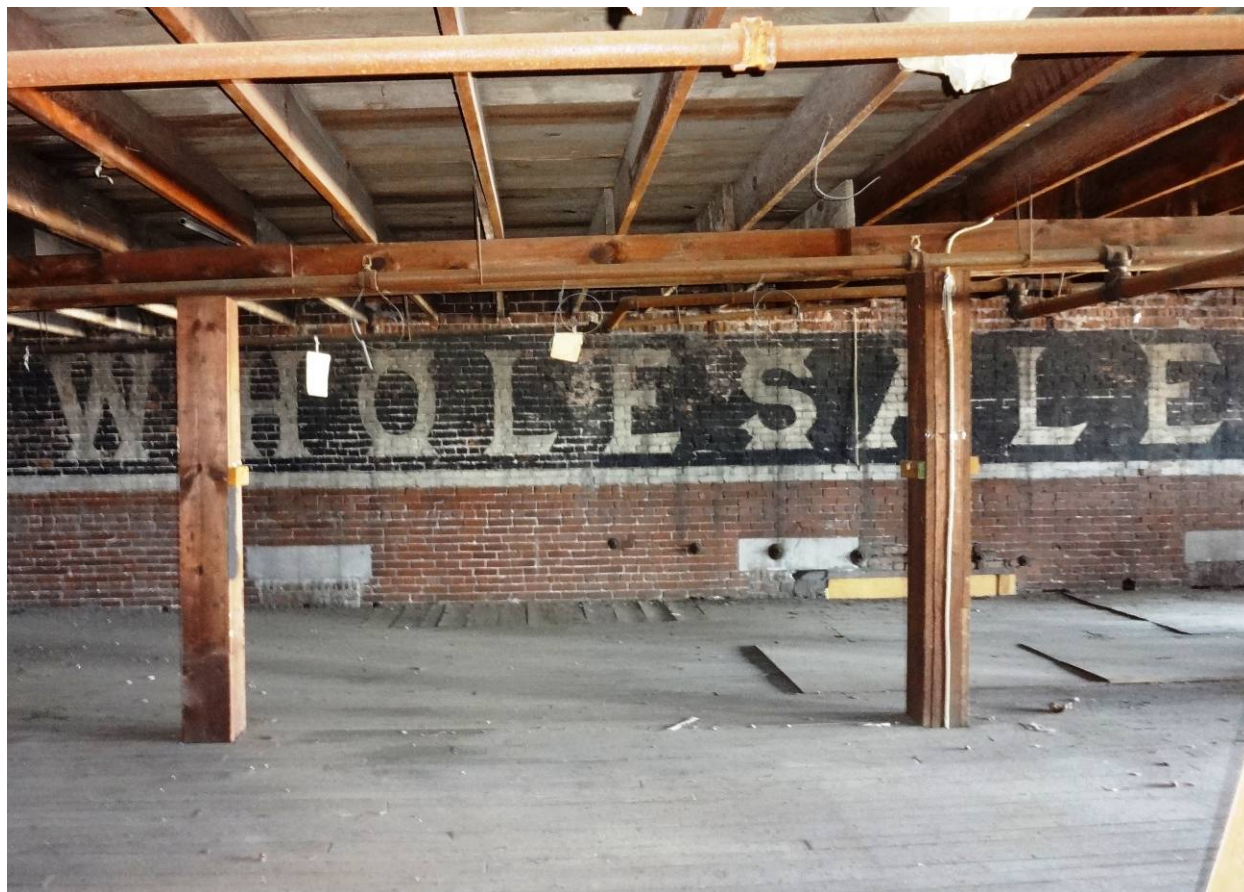
Photo 16. South third floor, looking north. (Original outside wall.)
