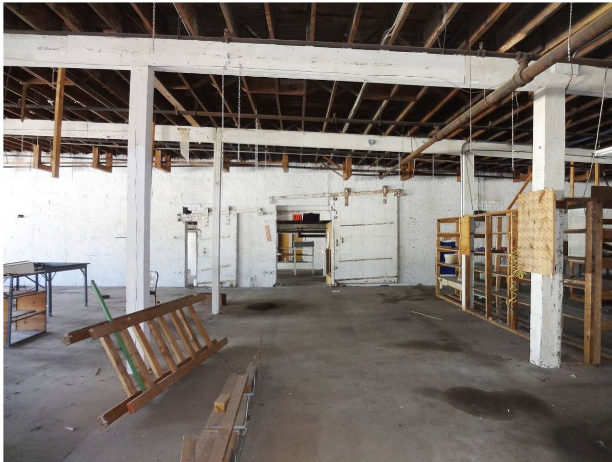
Photo 13. North second floor, looking south.
