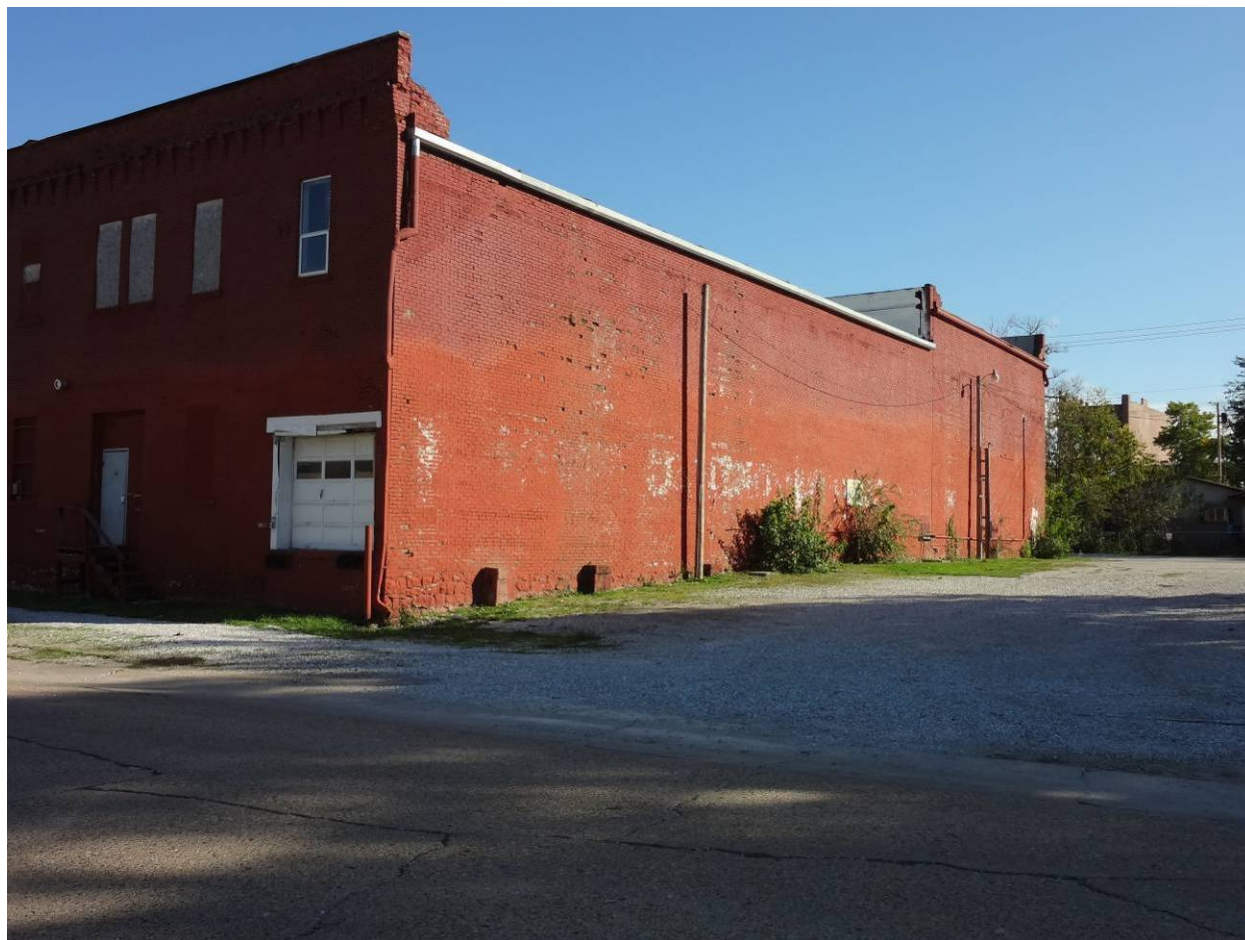
Photo 8. Back (west) wall, from the north.
