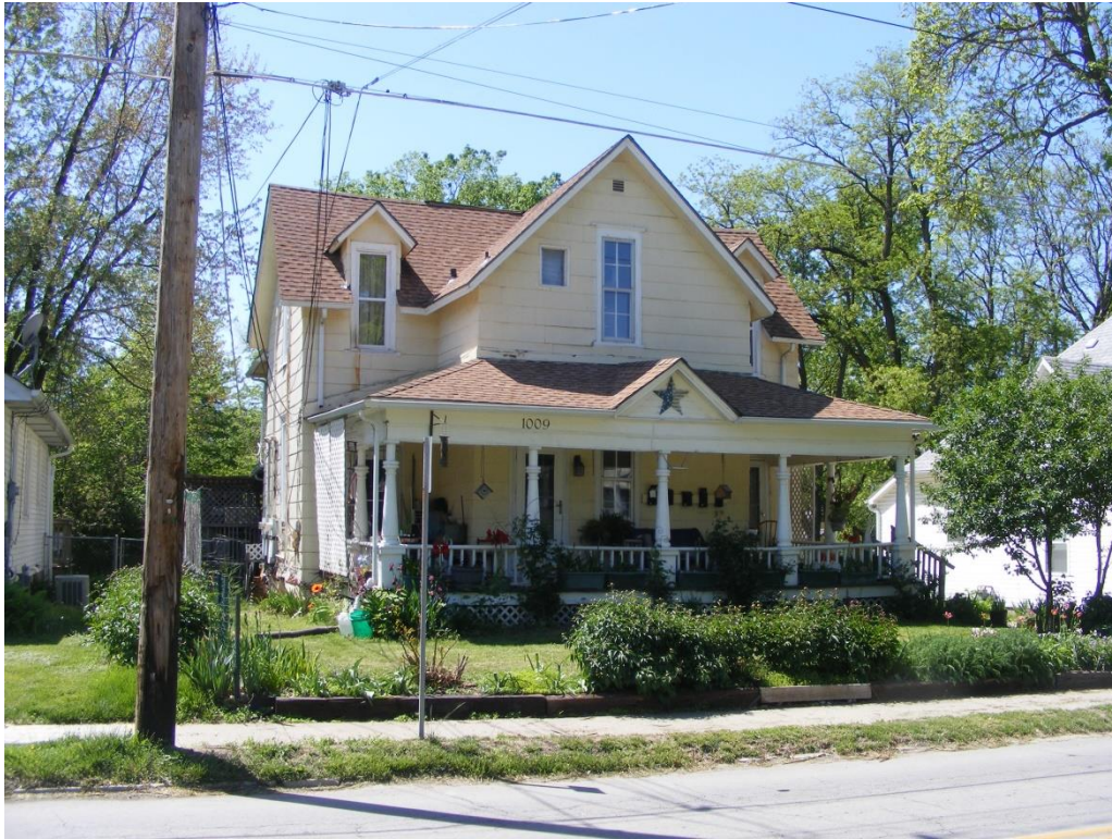
Figure 33. 1009 Range Line Street is one of two examples of the Queen Anne style in the survey area (Photo: Adam Flock, April 2019).
