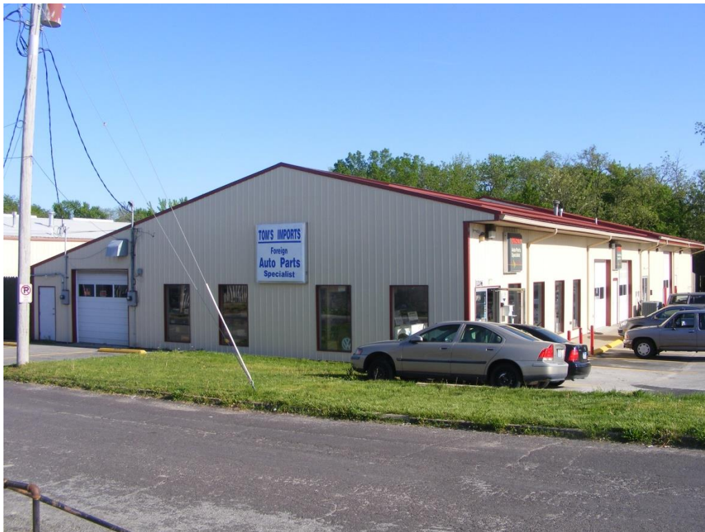
Figure 32. 1206 N. Coats Street is an example of a prefabricated warehouse-style building in the survey area (Photo: Adam Flock, April 2019).
