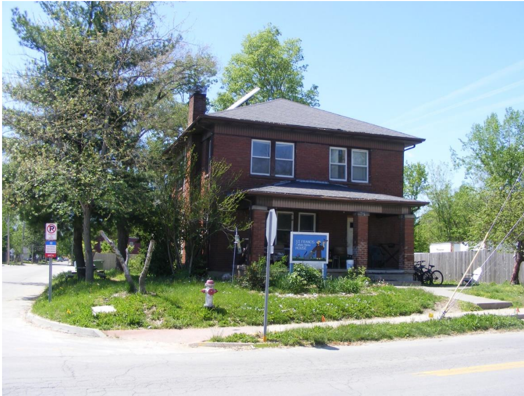
Figure 19. 901 Range Line Street is an American Foursquare style dwelling (Photo: Adam Flock, April 2019).
