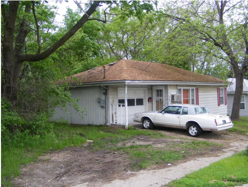
Figure 34. 1003 N. College Avenue is a Ranch style dwelling (Photo: Adam Flock, April 2019).
