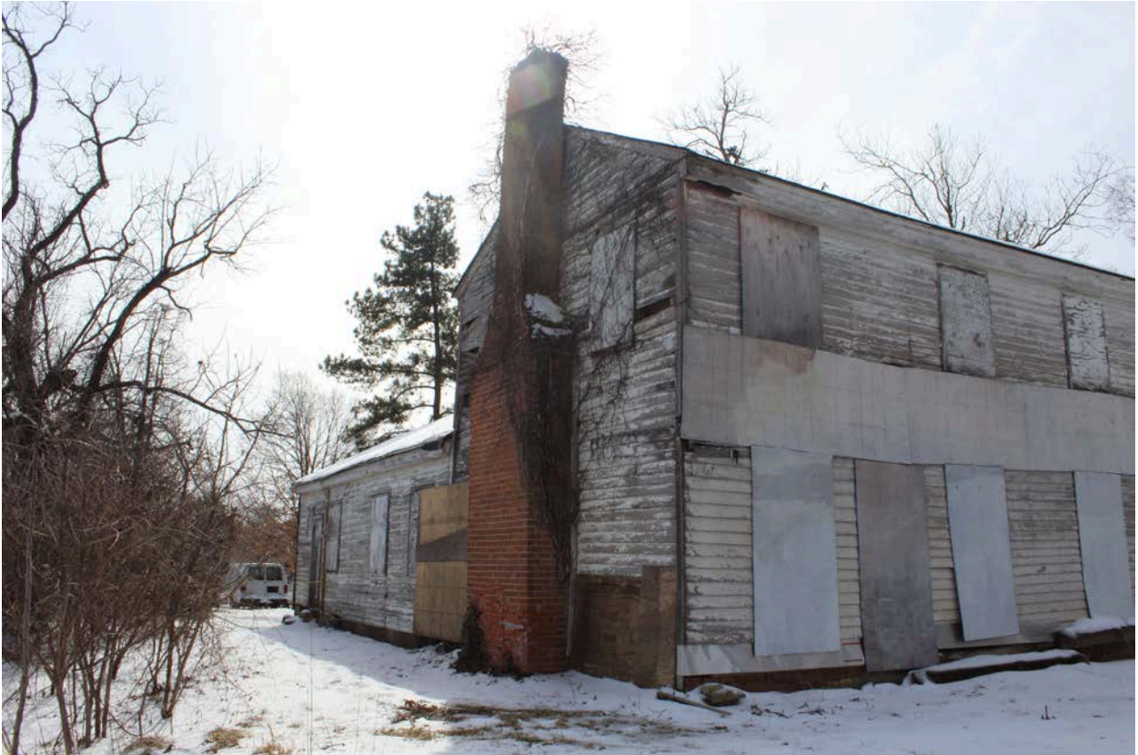
Henry Miller House, eastern elevation, February 2014
