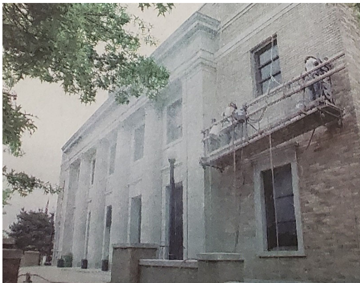
Figure 35: Photograph, 2000 Brick repointing during a 2000 renovation. (Joplin Globe)
