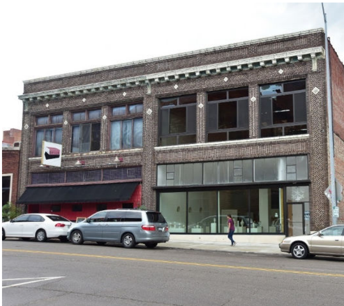
Figure 9. 1727-29 McGee Street (Resource #5). Photo by Brad Finch, 2017.
