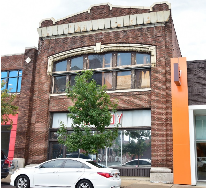
Figure 14. 1817 McGee Street (Resource #10) has a brick façade with terra cotta detailing. Photo by Brad Finch, 2017.
