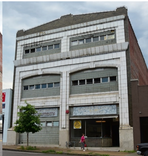
Figure 10. 1827 McGee Street (Resource #13). Photo by Brad Finch, 2017.
