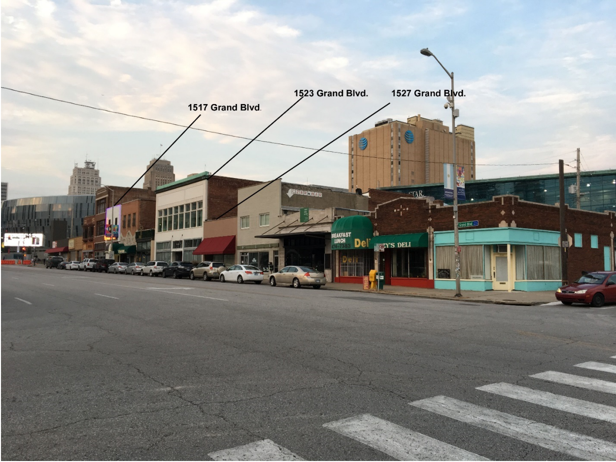
Figure 16. The buildings at 1517 Grand Boulevard, 1523 Grand Blvd., and 1527 Grand Boulevard. The Midtown Survey Final Report. Kansas City, Jackson County, Missouri (1981-85) identified these buildings as transportation related automobile properties. Photo by Sophie Roark, 2017.
