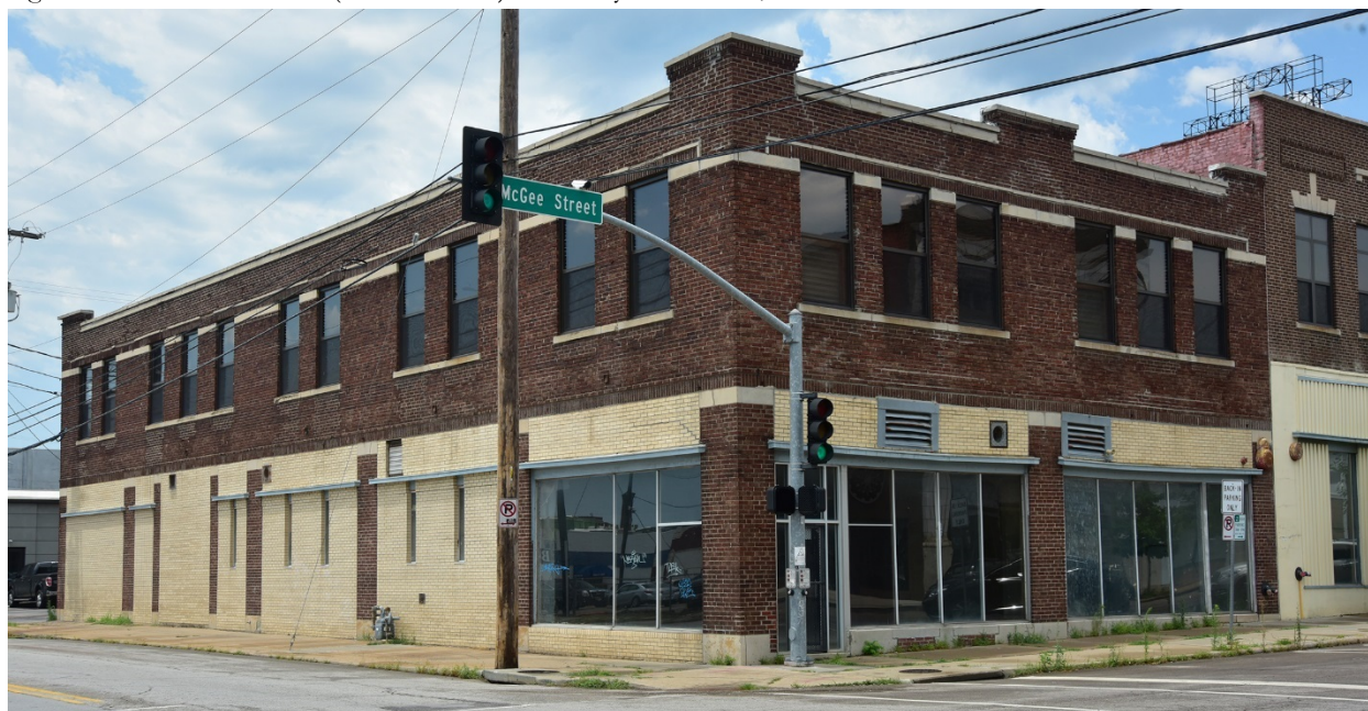
Figure 8. 1832 McGee Street (Resource #28). Photo by Brad Finch, 2017.
