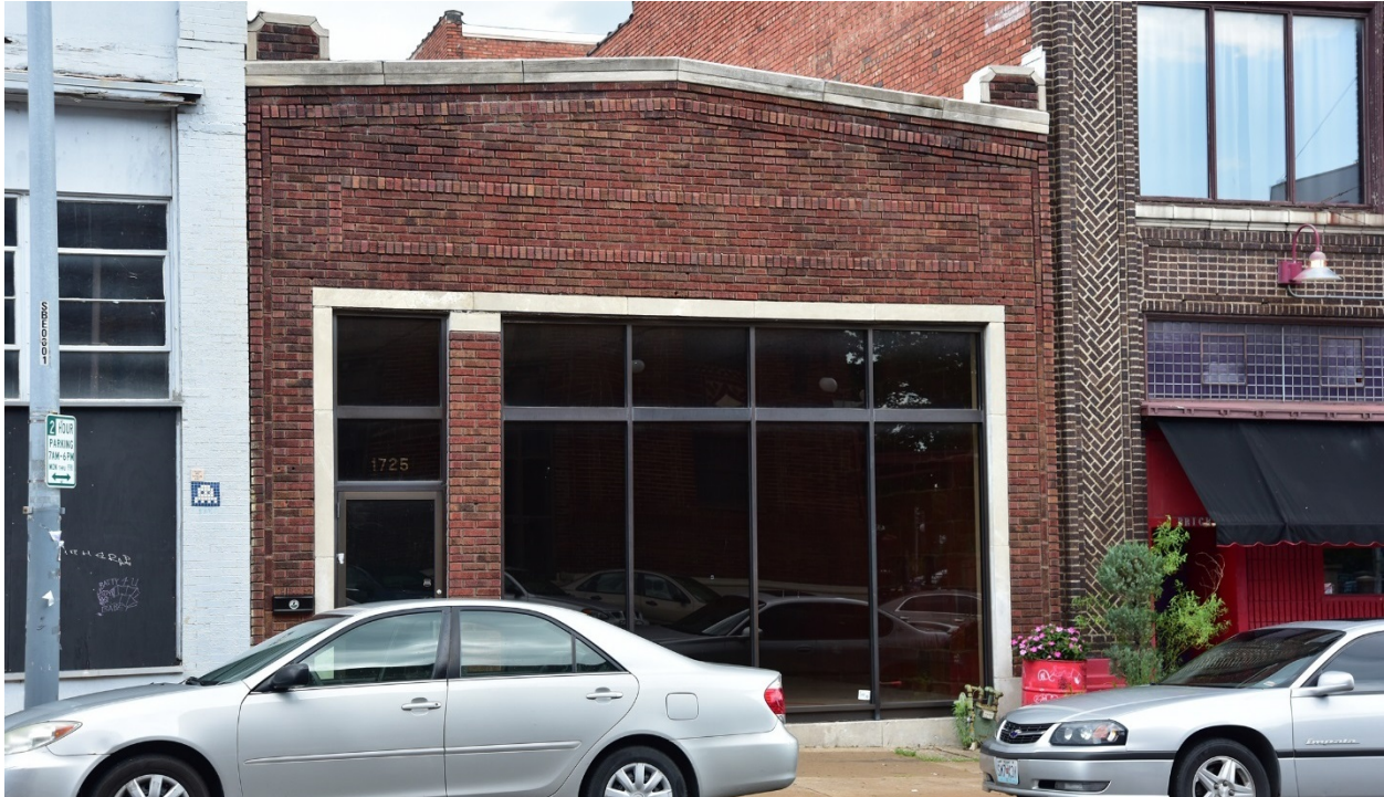
Figure 7. 1725 McGee Street. (Resource #4). Photo by Brad Finch, 2017.
