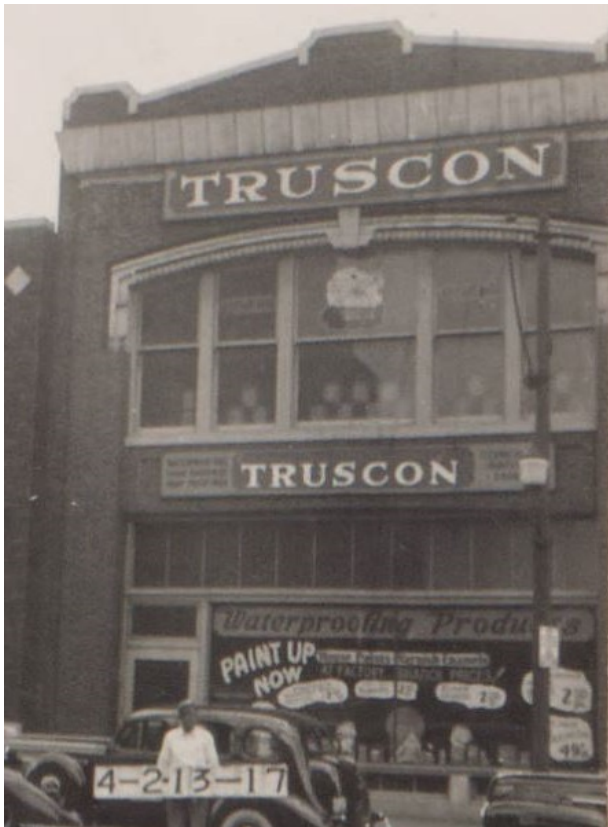
Figure 15. 1817 McGee Street (Resource #10) in 1940. Source: Kansas City 1940 Tax Assessment Photographs Missouri Valley Special Collections, Kansas City Public Library, Kansas City, Missouri.
