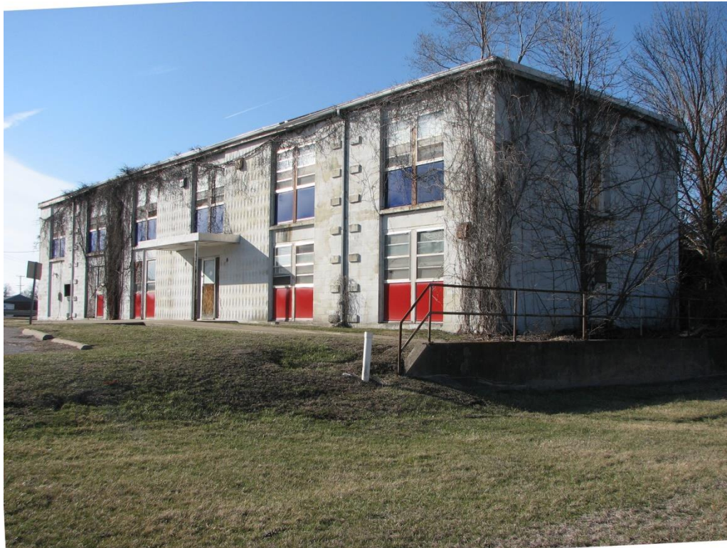
Figure 46. Locally known as “The Beanery,” 244 N. Moulton was constructed c. 1960 and used by the railroad company for employees who were stationed temporarily or overnight in Moberly (Photo: Ruth Keenoy, 2018).
