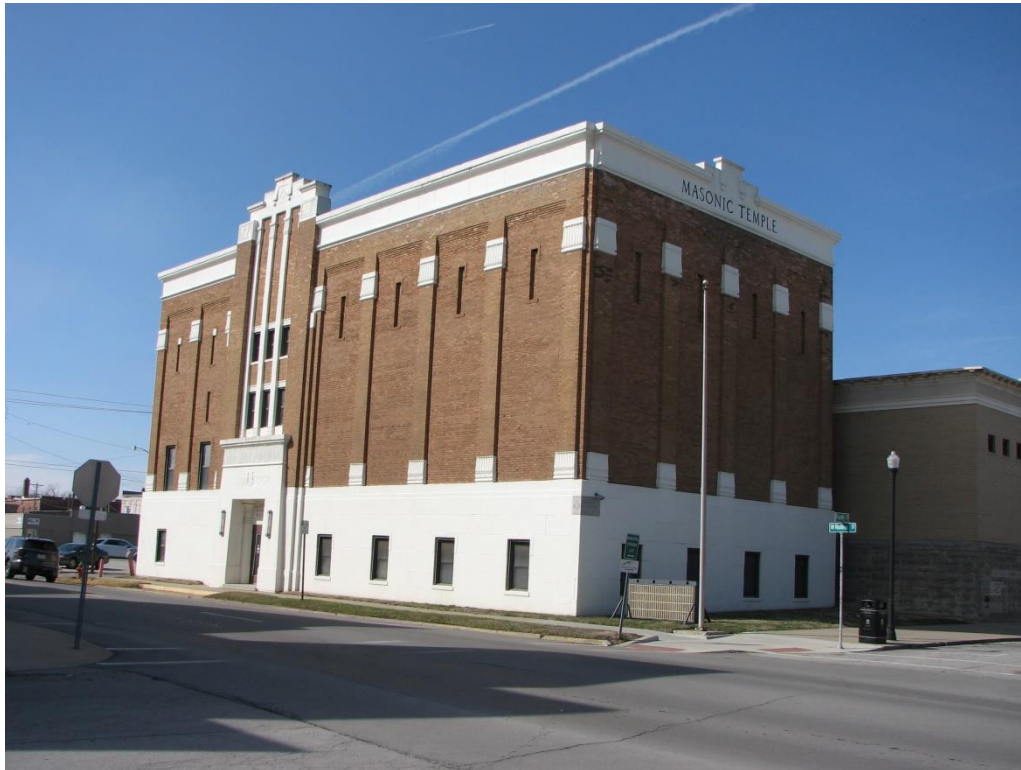
Figure 47. 401 W. Rollins Street is individually eligible under Criterion C: Architecture. View is northwest (Photo: Ruth Keenoy, 2018).
