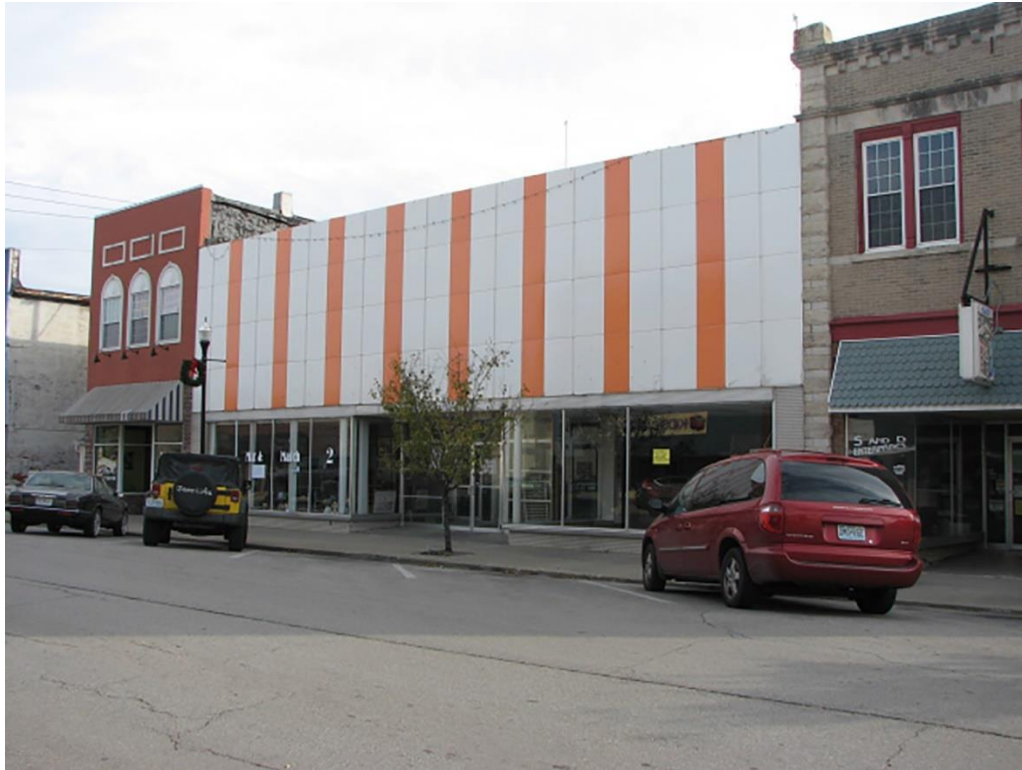
Figure 30. 416 W. Reed Street, which formerly held J.C. Penney's, was clad with a modern storefront in the 1960s (Photo: Ruth Keenoy, November 8, 2017).
