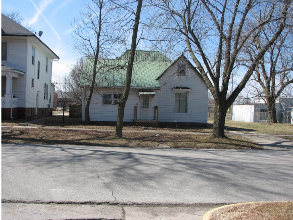
Figure 54. Although 323 N. Williams Street has been modified with a porch enclosure, the dwelling retains evidence of its Folk Victorian influence through its 1.5-story gable and wing plan and Queen Anne-influenced windows. View is west (Photo: Ruth Keenoy, 2018).
