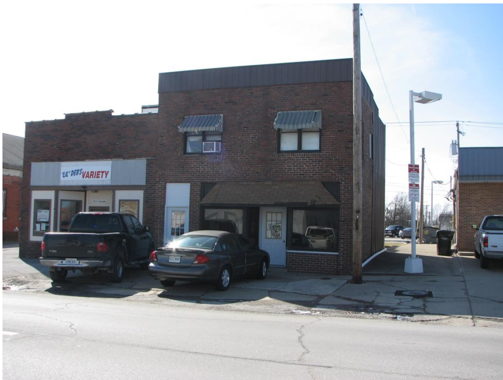
Figure 40. 113 S. Williams Street (left) and 111 S. Williams Street (right) were constructed in 1929. These buildings share a common wall and may be individually eligible under Criterion A (commerce/industry). View is southwest (Photo: Ruth Keenoy, 2018).
