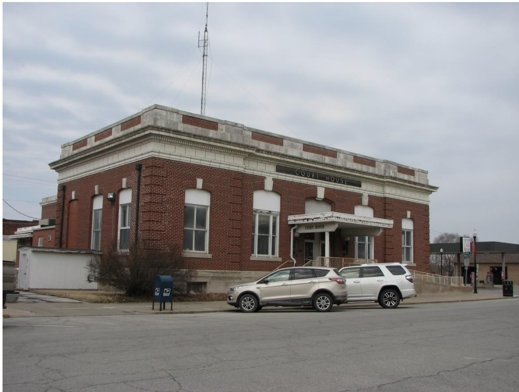
Figure 44. 223 N. Williams Street was originally a post office, converted for use as city offices and a court house. View is northwest (Photo: Ruth Keenoy, 2018).
