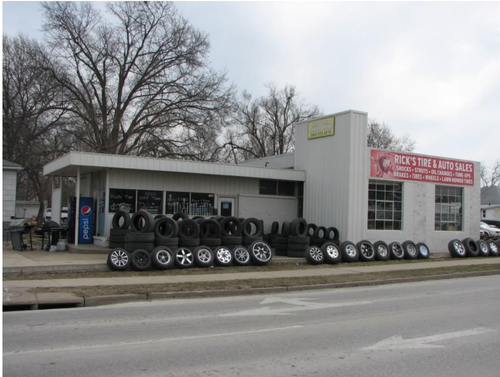
Figure 63. 120 S. Morley Street would contribute to an auto-related district recommended for properties at the intersection of Morley and E. Rollins Streets (Photo: Keenoy, March 2018).
