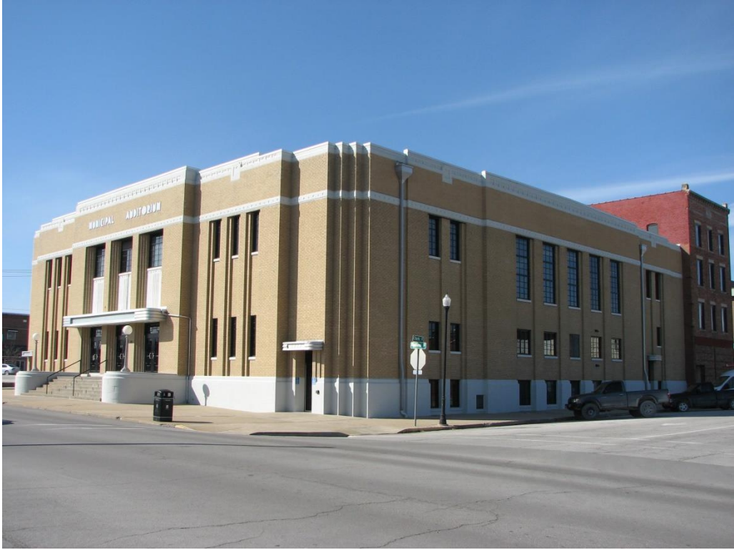
Figure 37. 109 N. Clark Street, view is northwest. The property is individually eligible under Criterion C (Architecture)
