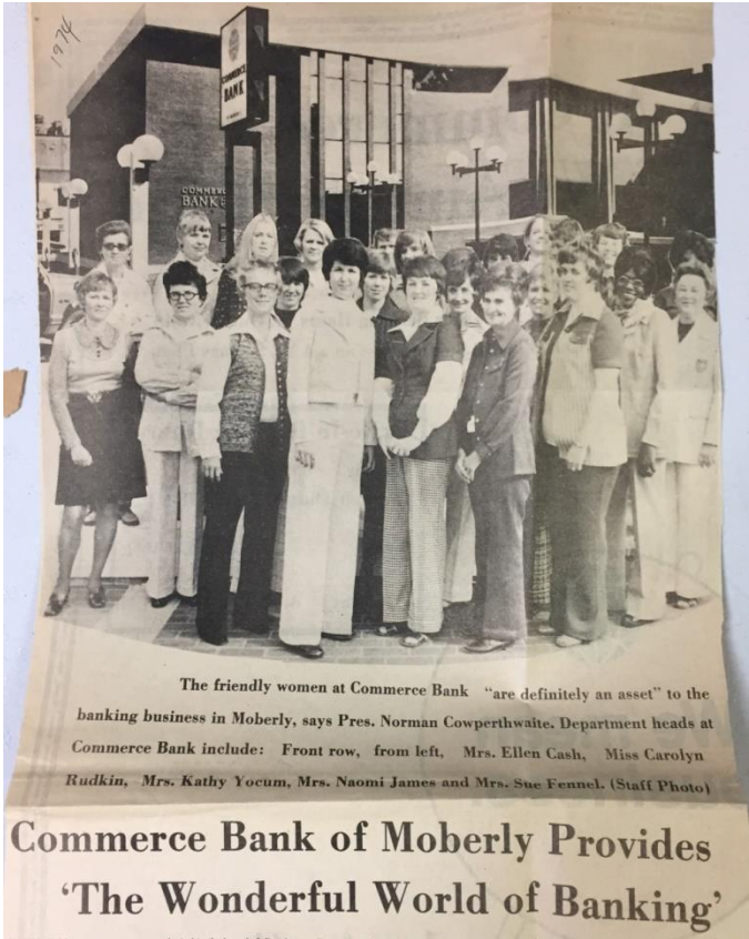
Figure 33. Commerce Bank at 208 W. Reed Street was constructed in 1970 and designed by Joseph Cleavinger. The building is recommended as individually eligible for its architectural significance and is included within the recommended downtown district boundary expansion area (Source: clippings, Randolph County Historical Society).
