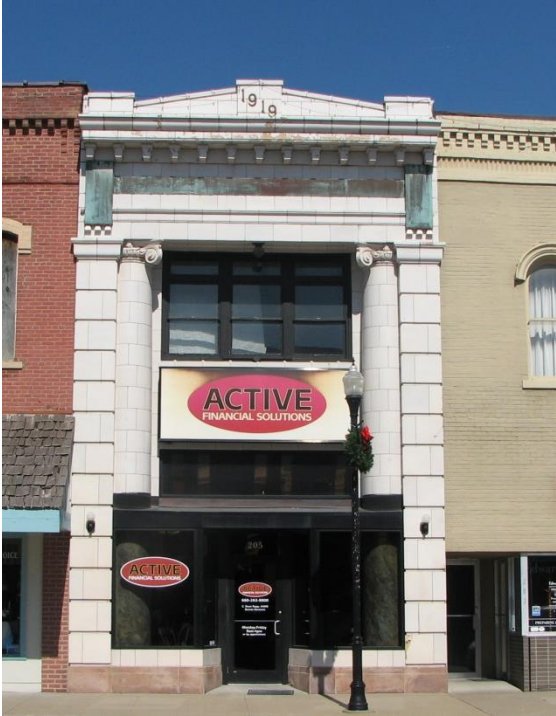
Figure 42, 205 W. Reed Street is a contributing property within Moberly’s 2012 Commercial Historic District that may be individually eligible for its architectural contributions (Photo: Ruth Keenoy, 2017). View is north.
