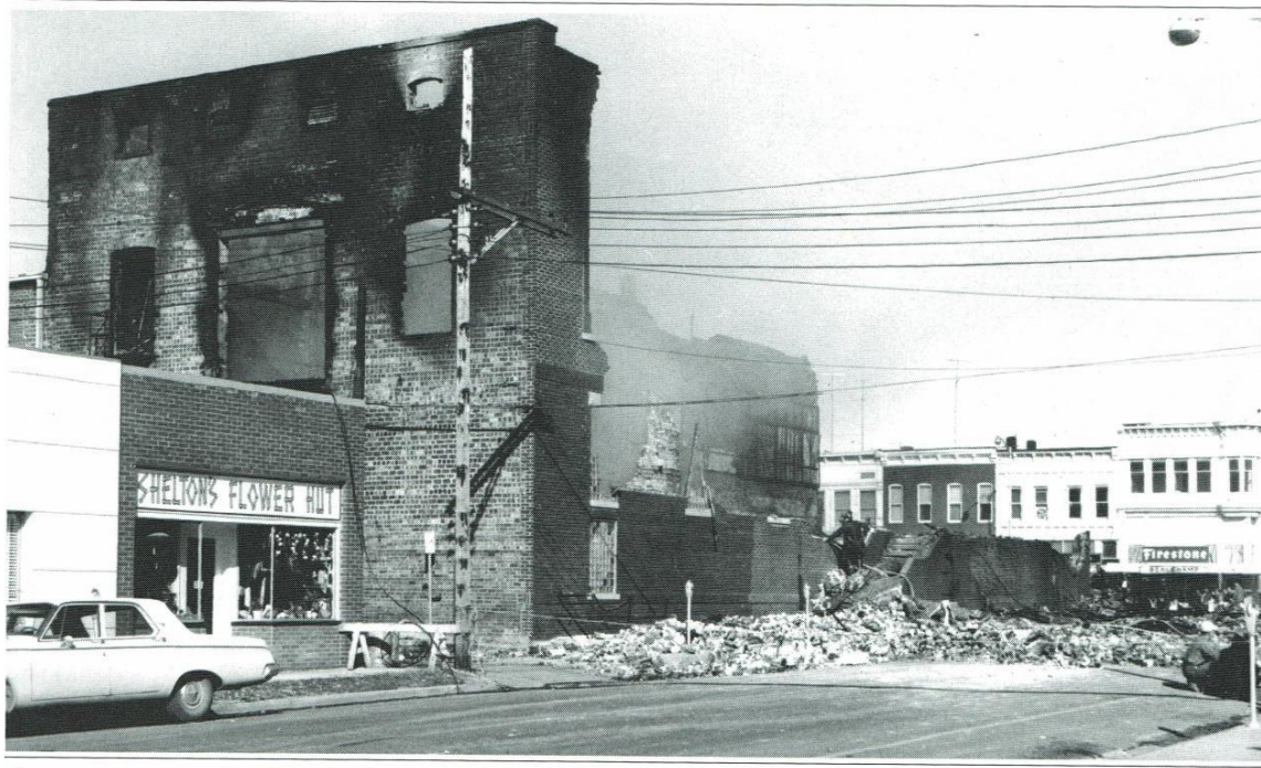
Figure 27. Fire in 1966 destroyed three buildings at the intersection of W. Reed and N. Fifth Streets (Source: Orton and Court, 106). View is northwest, taken from N. Fifth Street.
