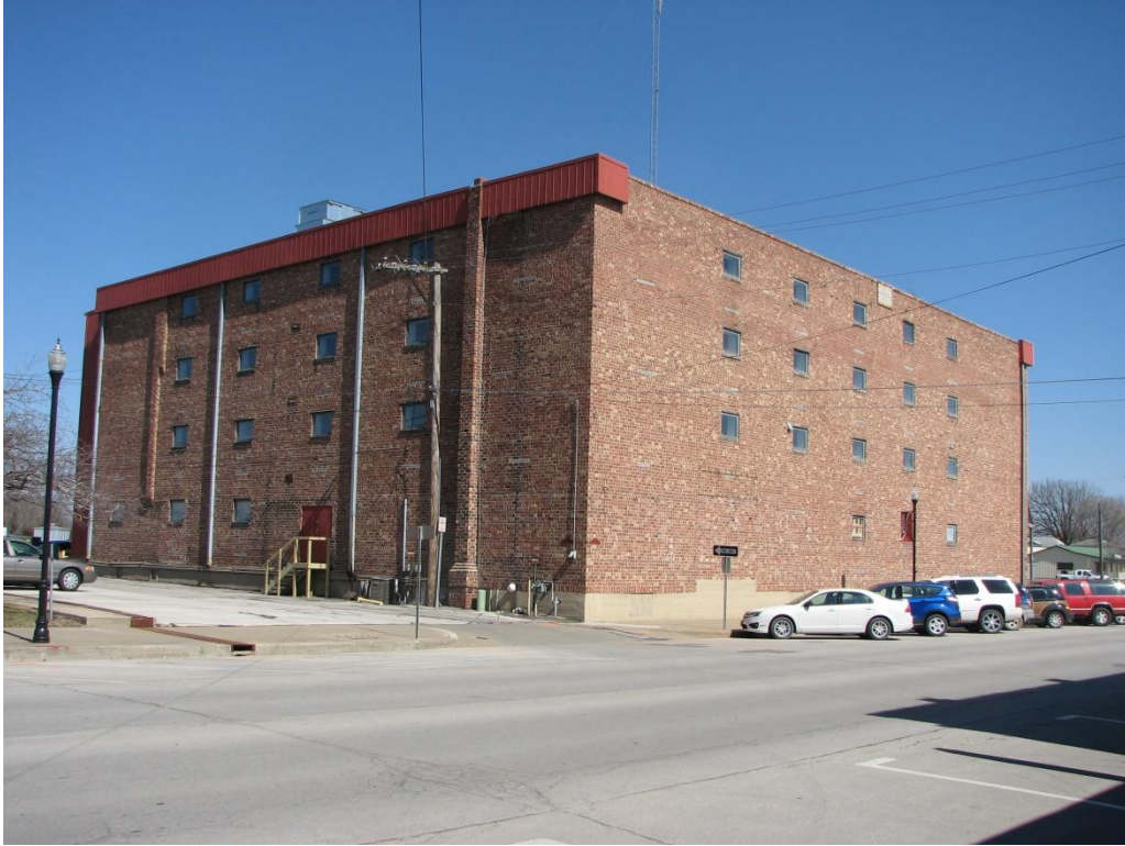
Figure 61. 101 W. Coates Street was constructed in 1919 as a grocery warehouse. View is northeast (Photo: Ruth Keenoy, 2018).
