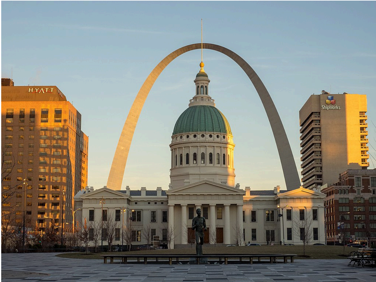
Figure 6: Old Court House, St. Louis, MO. Source Wikimedia—facing east.
