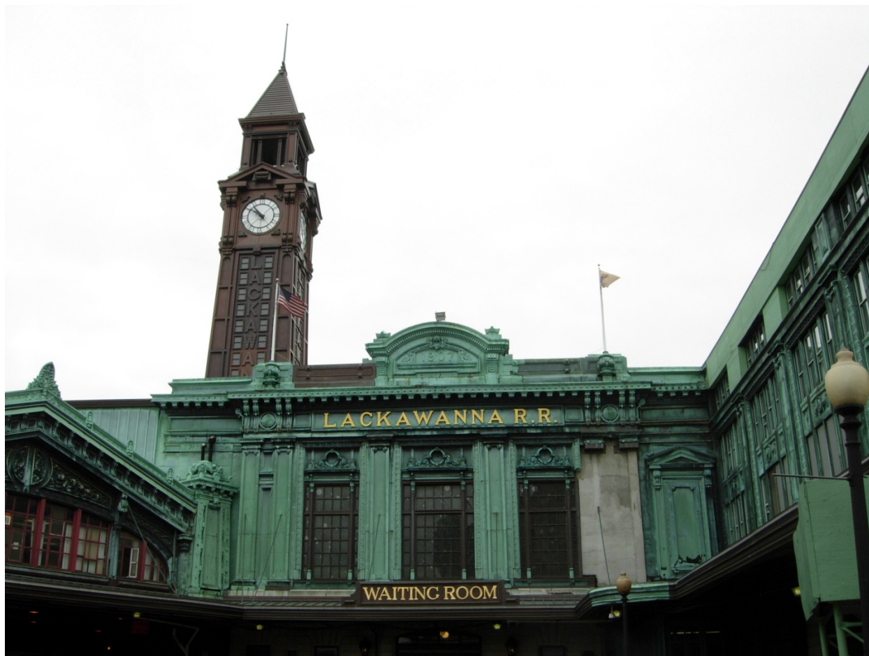
Figure 7: Hoboken Terminal, Hoboken New Jersey, source Larry Peters
