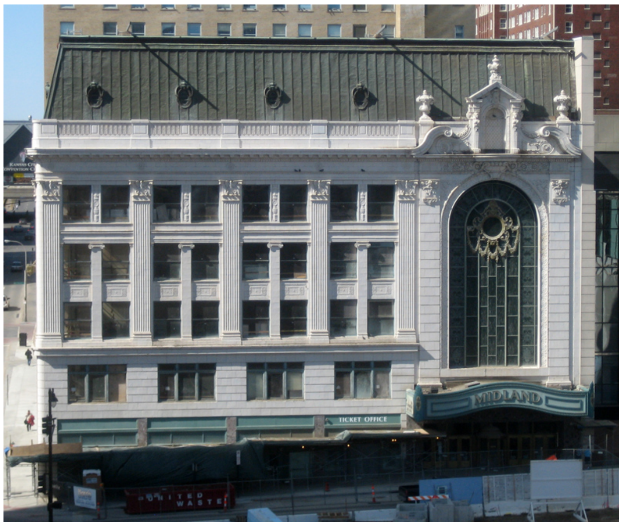
Figure 2: The Midland Theater Building, Kansas City, MO. Copper Mansard and Storefront Surrounds, Wikimedia
