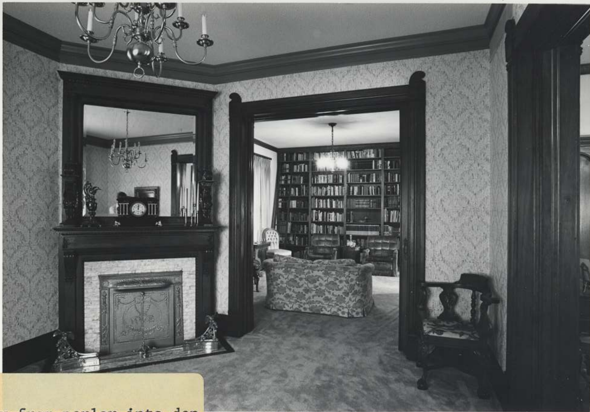
View from parlor into den, looking south
