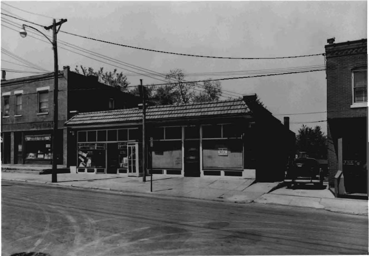
Goldstein's Piggley Wiggley Grocery Store, 741 and 743 Marshall Avenue, built 1927. Photograph taken 1962, courtesy Bob Wood.
