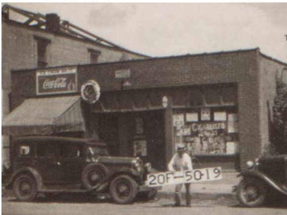
Figure 12. 8107 Woodland Avenue (The Paseo). 1940 tax assessment photograph.
