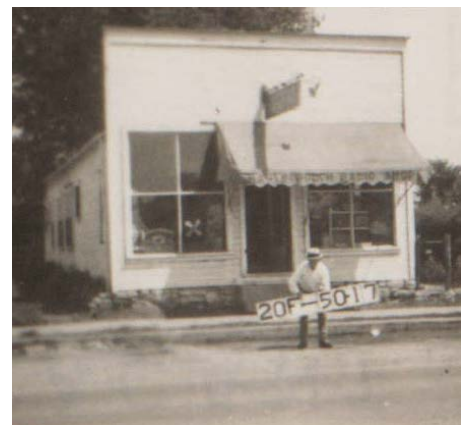
Figure 13. Radio Repair Shop, 8115 Woodland Avenue (The Paseo). 1940 tax assessment photograph.
