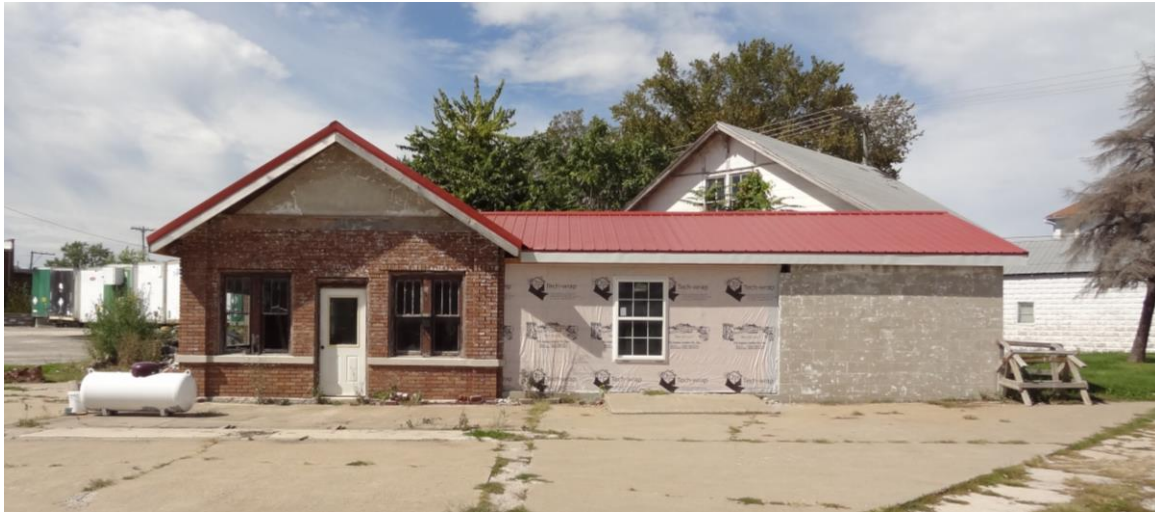
Figure 13. 211 E. Bourke St. (MC-AS-001-012) was constructed as an automobile service station.
