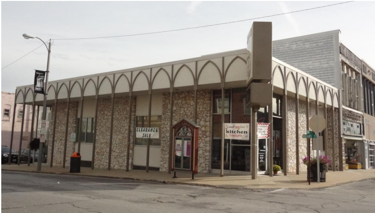
Figure 36. Macon Building and Loan Association (MC-AS-001-097), 101 Vine St., constructed in 1967.
