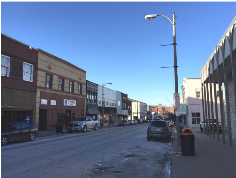
Figure 26. Streetscape looking north along N. Rollins St., part of potential historic district.
