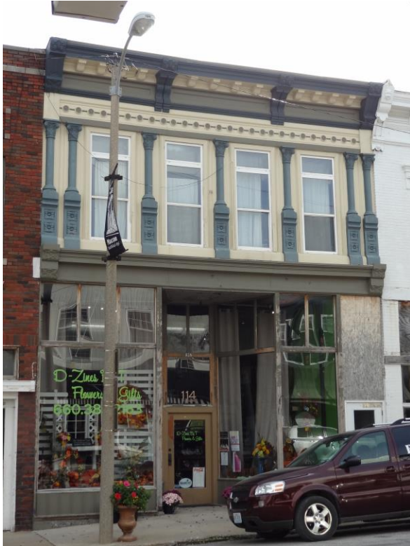
Figure 18. Historic Italianate features are retained on the upper facade of 114 N. Rollins St. (MC-AS-001-044), constructed c. 1890.
