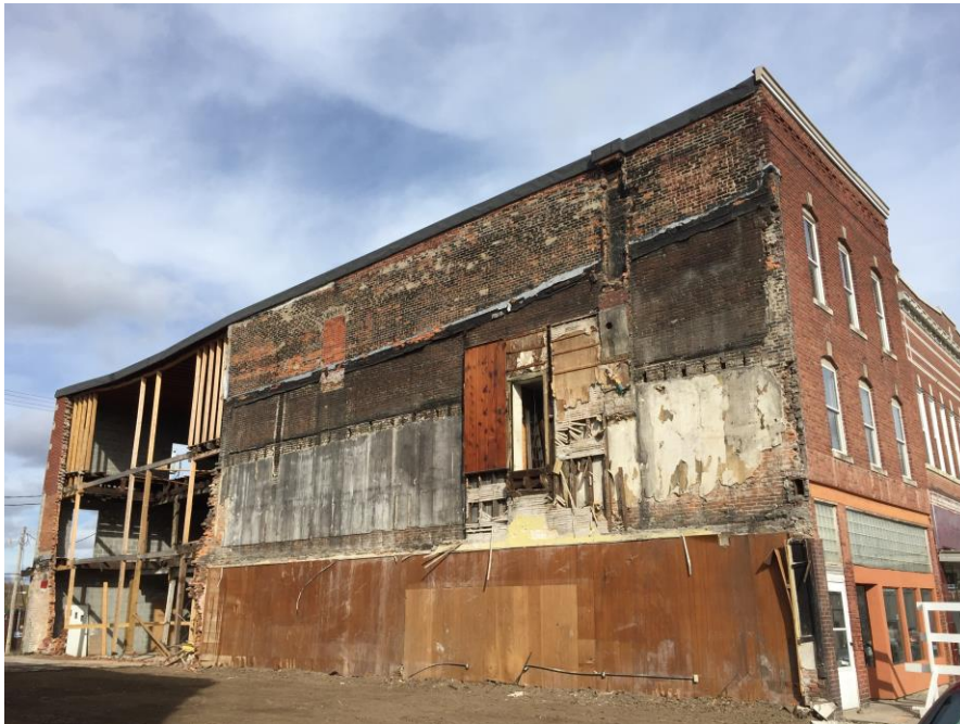
Figure 15. The parcel at 121 Vine Street after demolition (MC-AS-001-114).
