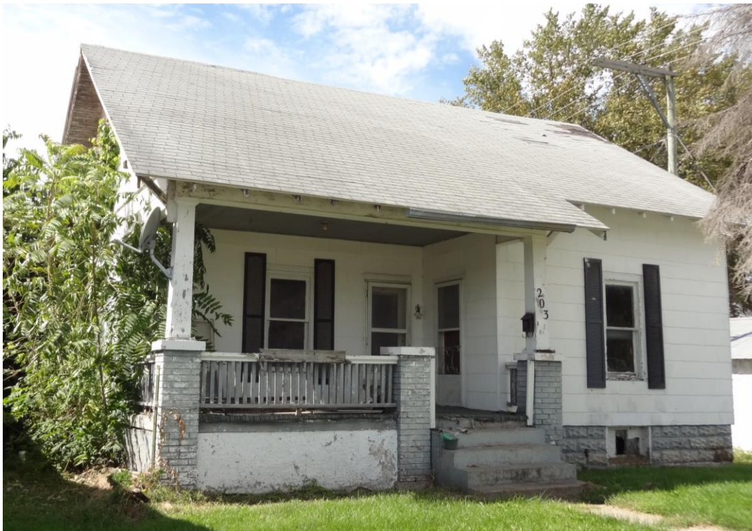
Figure 14. Single-family residence at 203 N. Rutherford St. (MC-AS-001-095).
