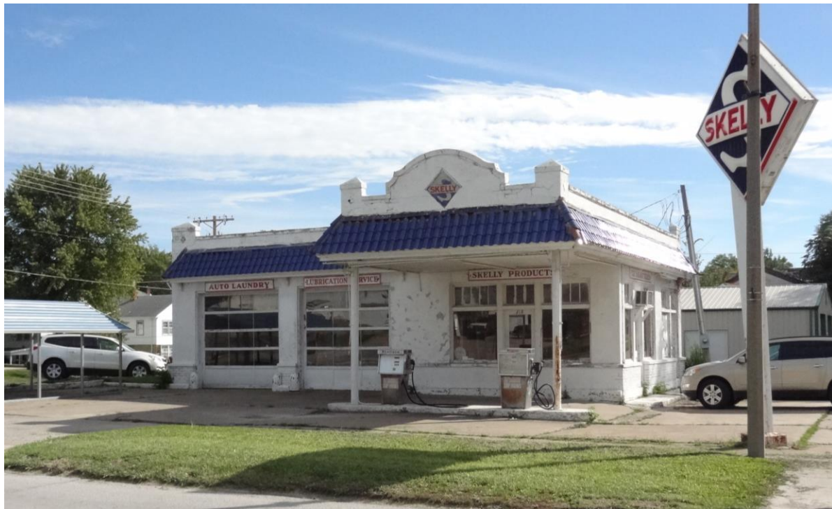
Figure 38. Skelly Oil Company Service Station (MC-AS-001-092), 218 N. Rubey St., constructed c. 1925.
