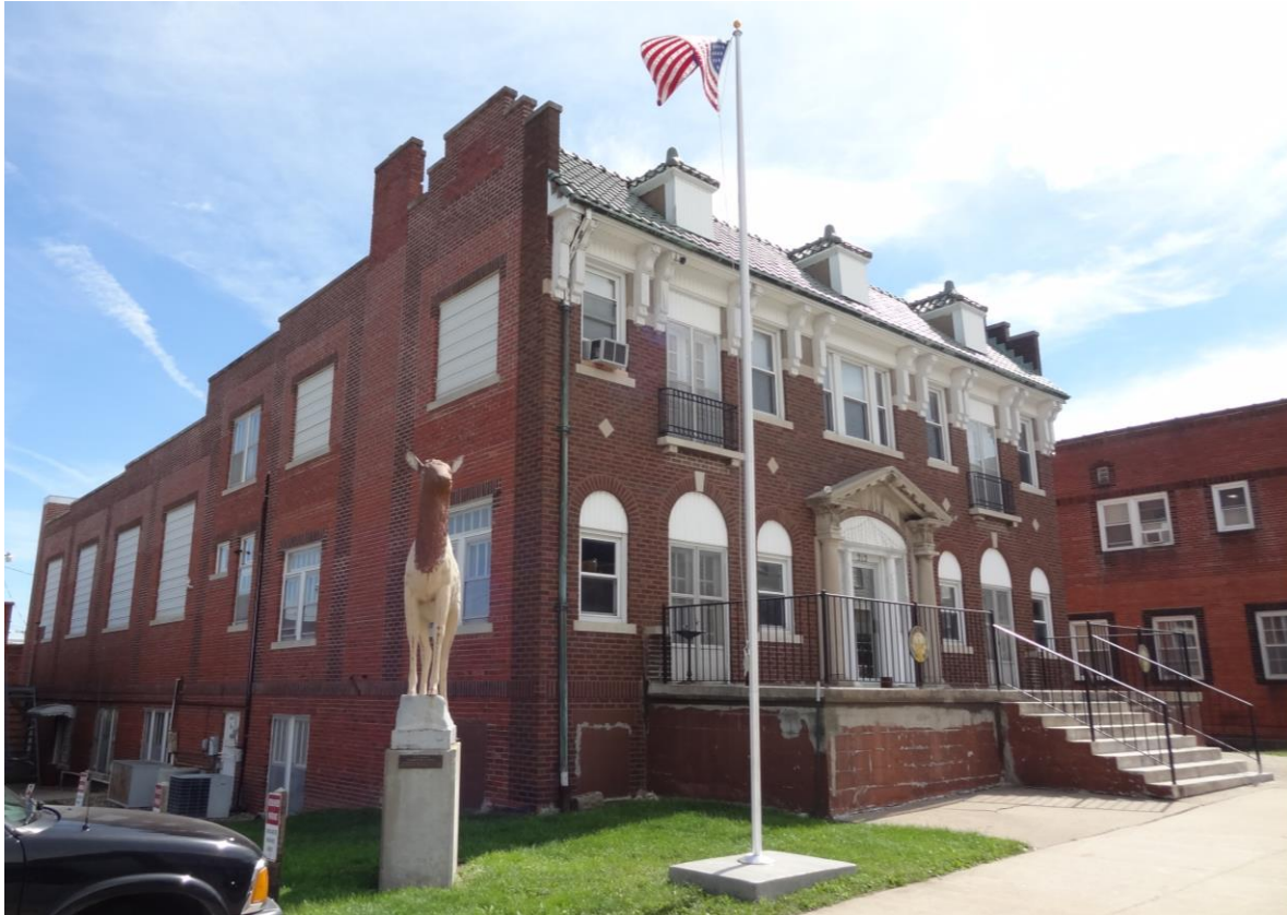
Figure 35. Elks Lodge #999 (MC-AS-001-058), 212 N. Rollins St., constructed in 1922.
