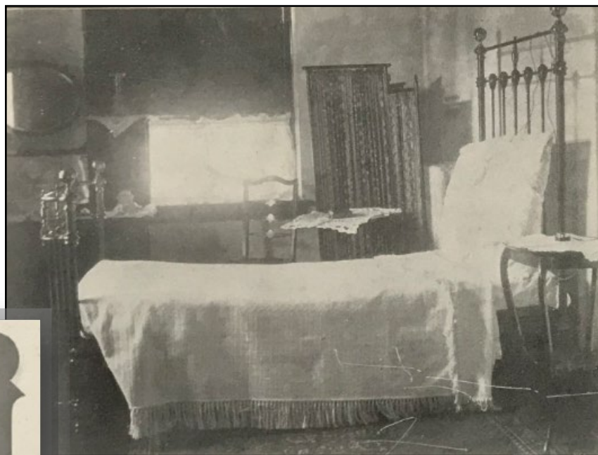
Figure 8.6: Period photographs of patient rooms in new addition, circa 1901. Source: Concordia Historical Society photograph file.
