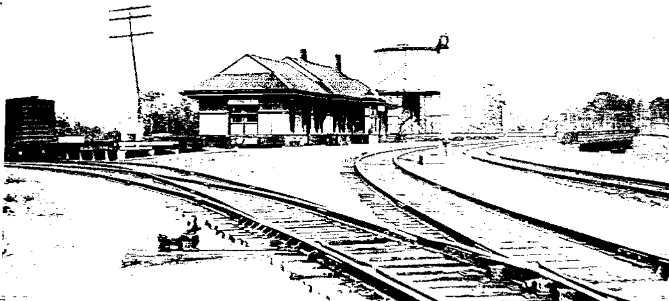
GOLF MUELLER + CHIC DEPOT ALTON, MISSOURIA - SHOWING WATER TANK + CRANES MAY 1941
