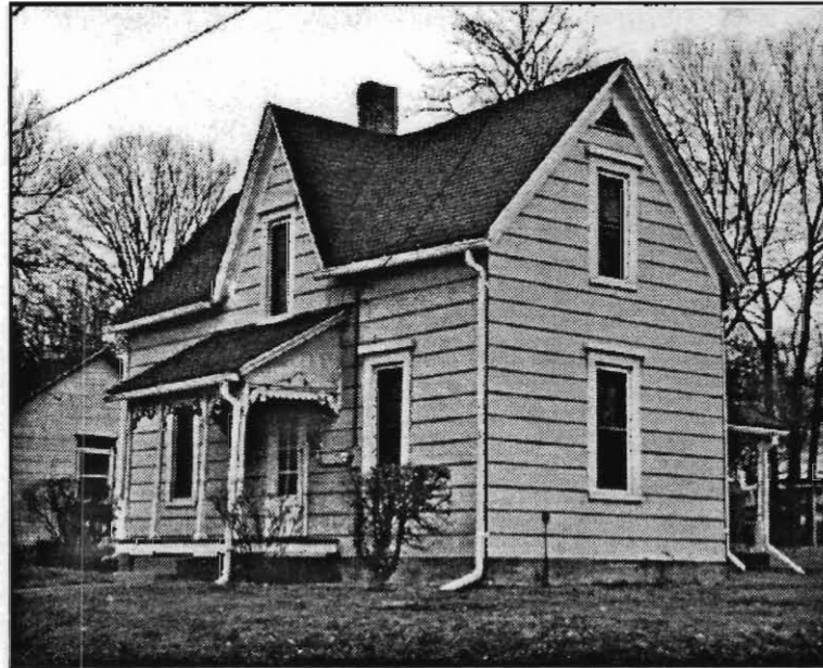
Asbestos siding on 403 N. Prairie, with shading to represent clapboards.
