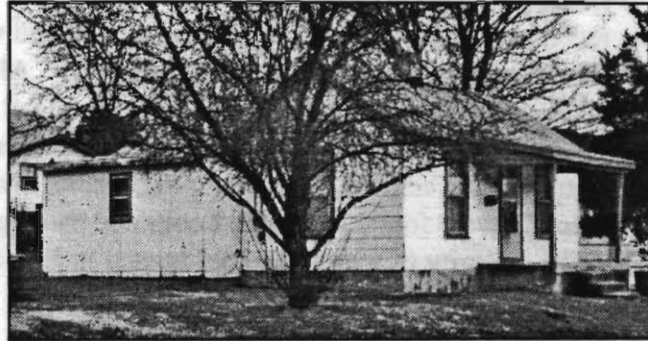
Additions to the rear of this hall & parlor at 315 Prairie do not detract from the original form of the residence on its primary facade.
