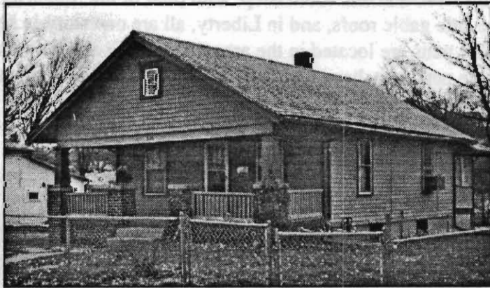
This bungalow at 336 Prairie retains its original siding and porch features.
