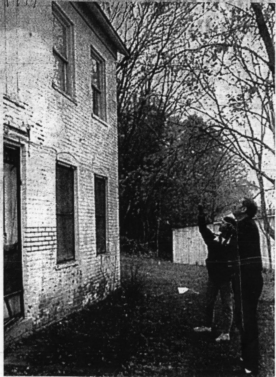
Debbie Sheals points out architecture of a LaGrange home to Lee Gilleard. Both are with the Missouri Department of Resources historical preservation program.
