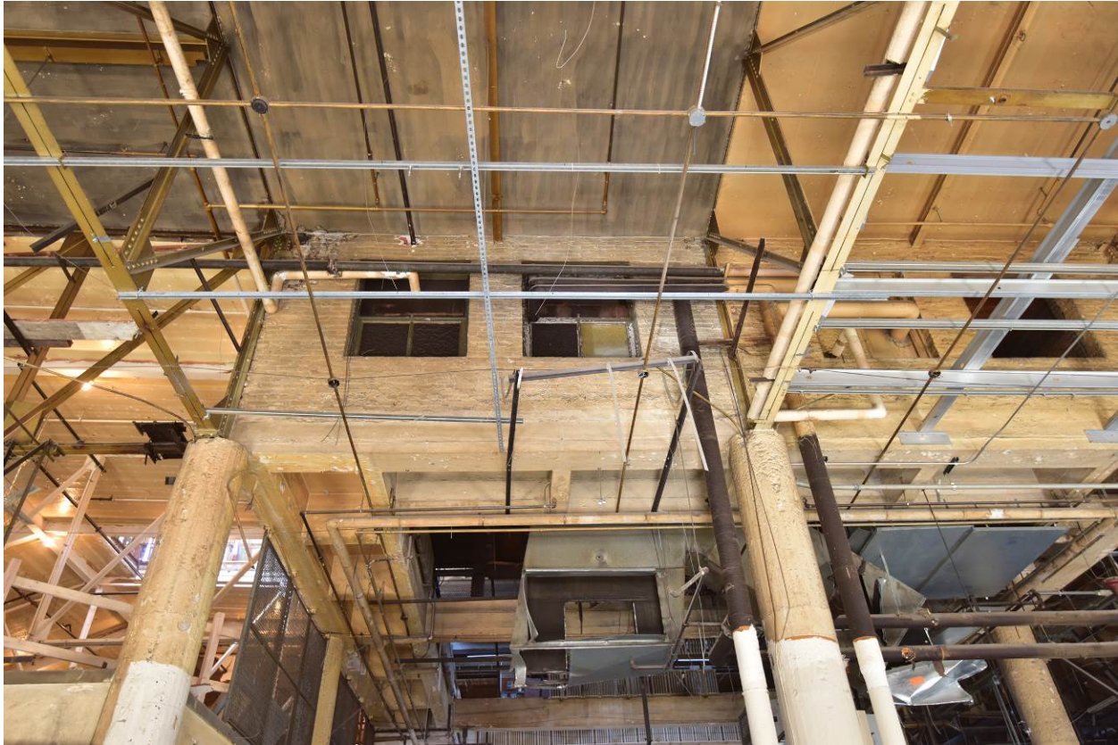
Figure 28. Enclosed skylight on 4 th floor of east wing. Brad Finch, 2017.
