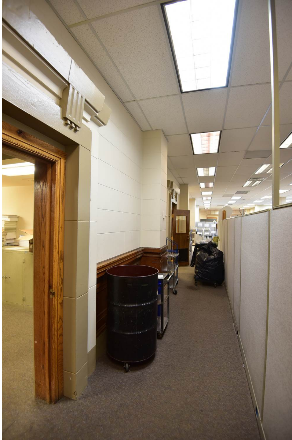
Figure 26. Historic door surround and scored plaster walls, 1 st floor of west wing. Brad Finch, 2017.
