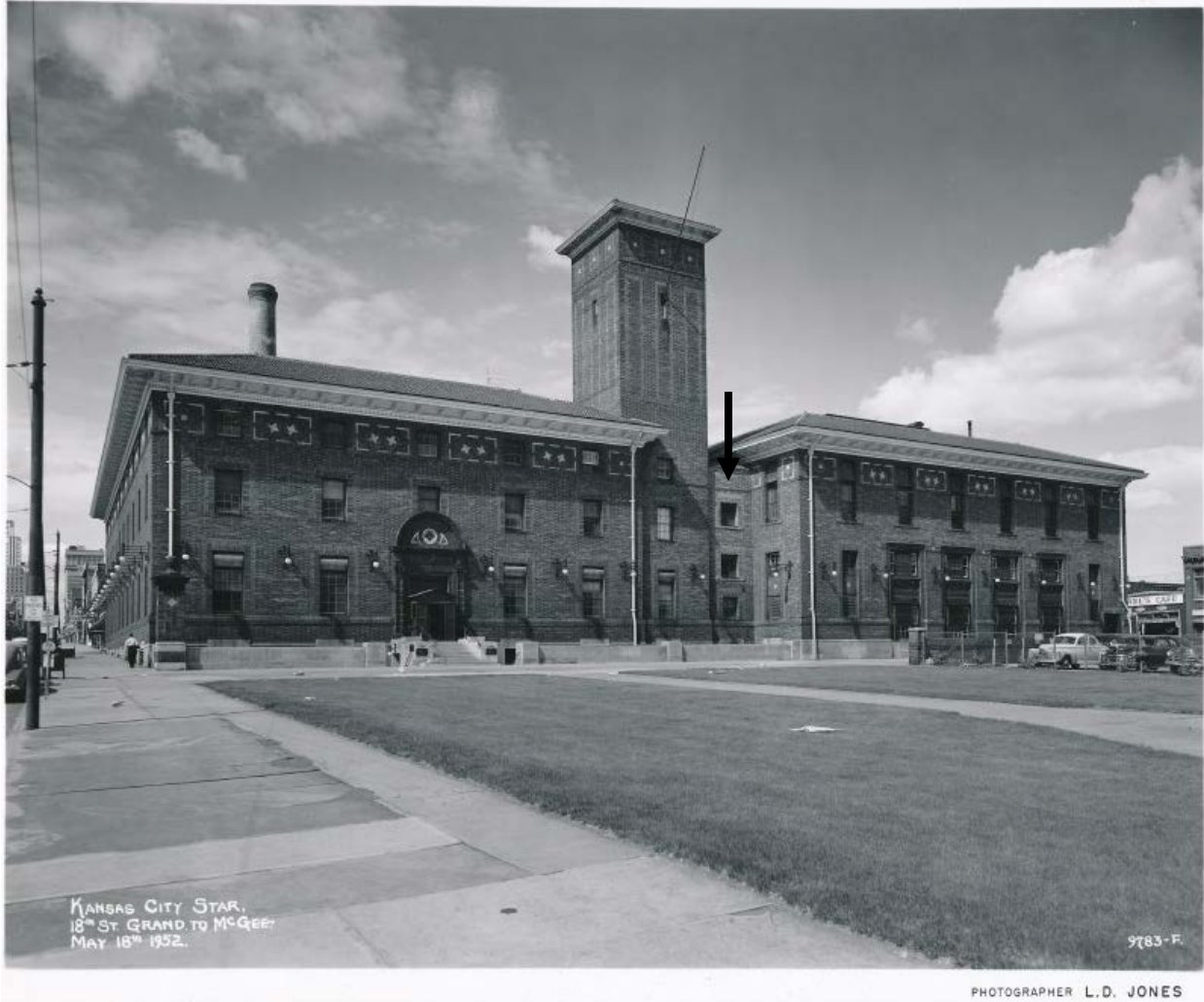
Figure 41. South elevation of Kansas City Star Building, May 18, 1952, L.D. Jones, photographer. Source: Wilborn Photo Studio. Note infilled area next to tower (see arrow) without fire escape.
