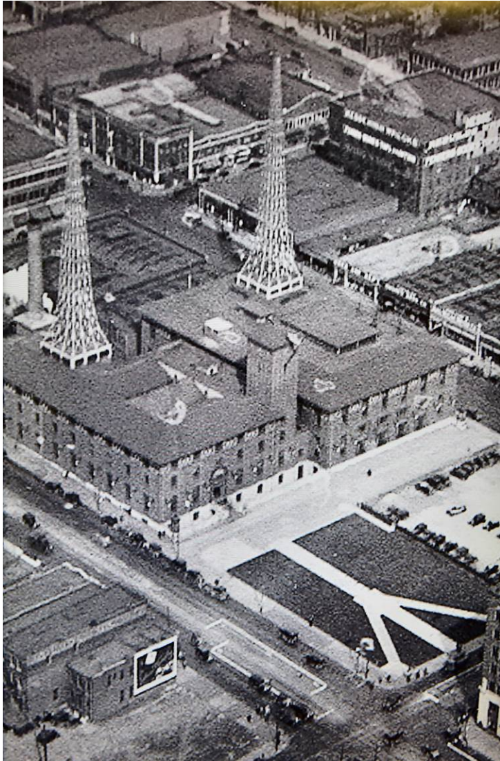
Figure 29. Aerial photo of broadcast towers, c. 1930. Kansas City Star Archives.
