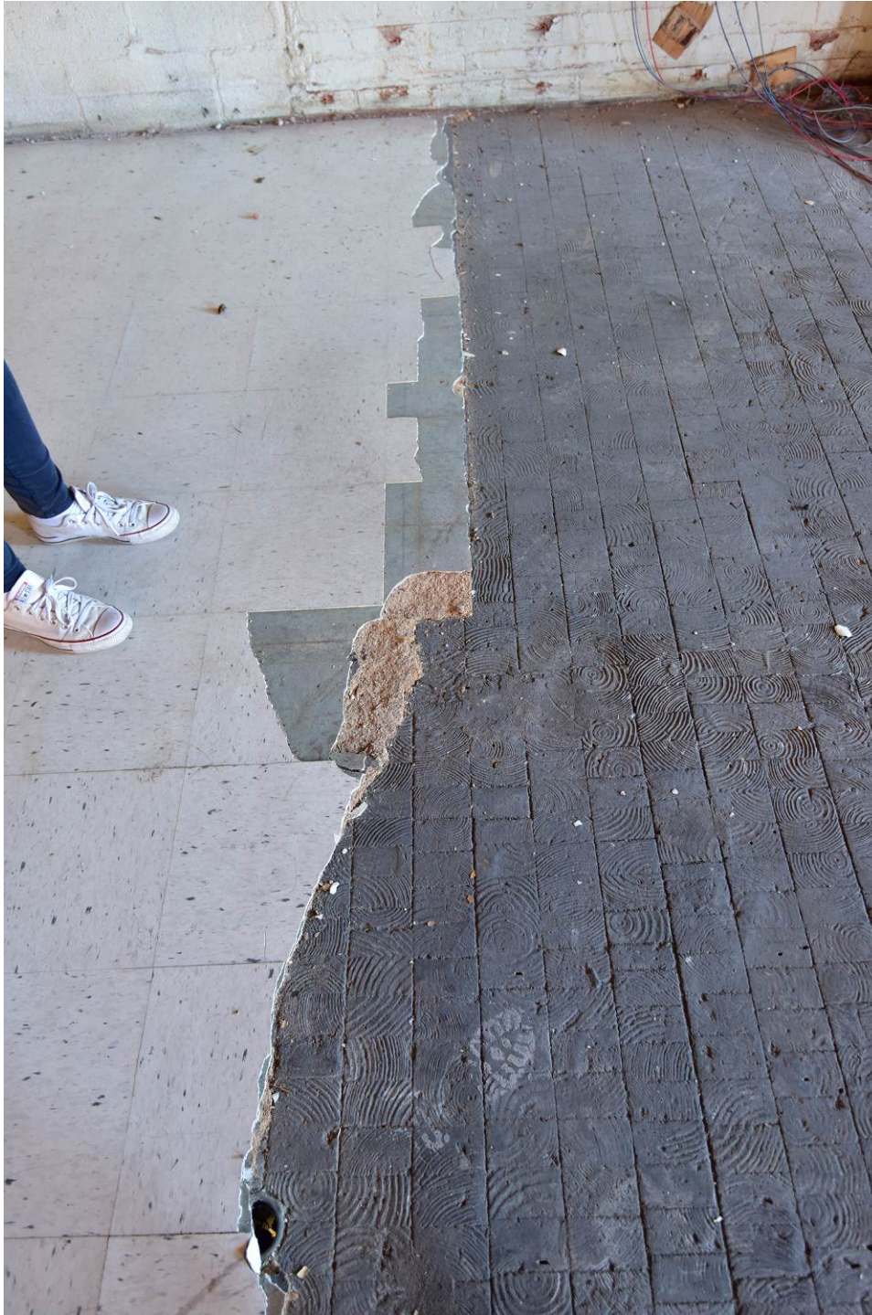
Figure 27. Historic wood block floor, 3 rd floor of east wing. Brad Finch, 2017.
