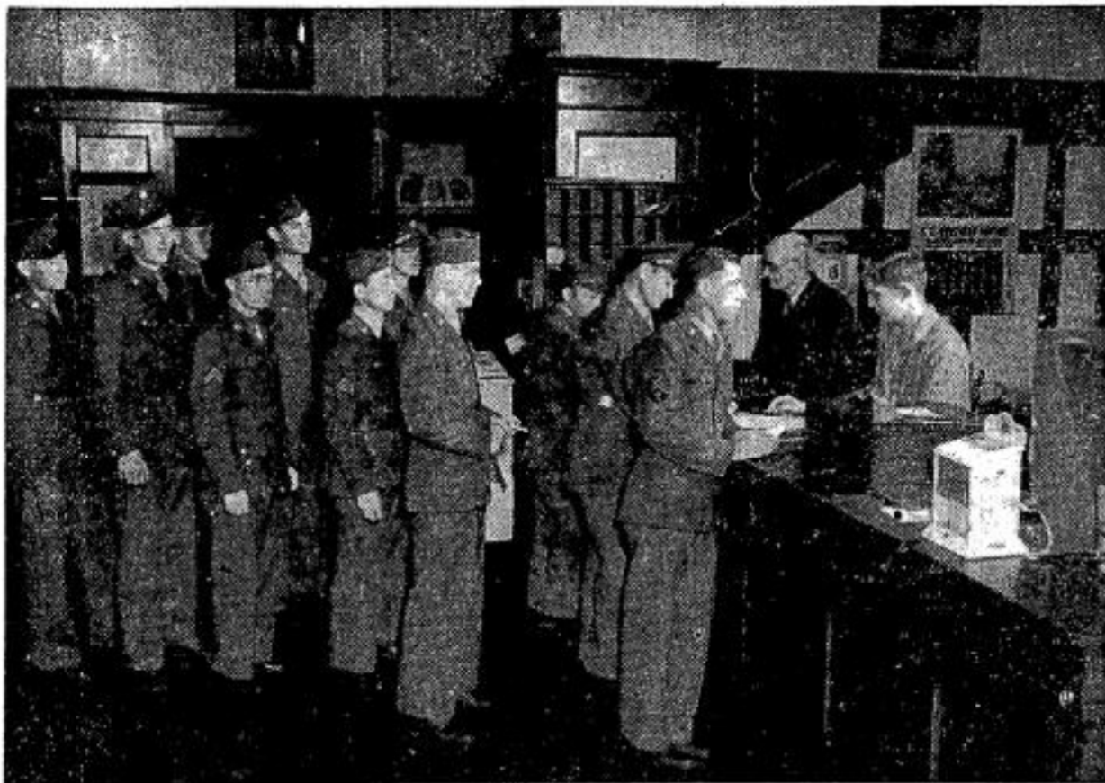
Figure 13. View of lobby in 1943, looking SSW and showing reception desk. Source: "An Inquirer Learns About the YMCA in Wartime," Joplin Globe (31 January 1943): E-5.
