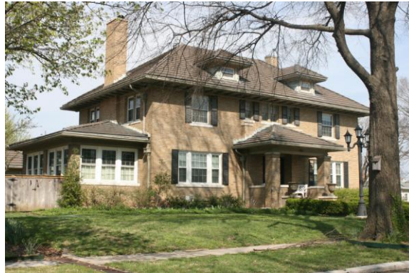
With its broad overhanging eaves and shallow pitched hipped roof with dormers, the 1922 Frank Childress House represents the Prairie style with Colonial Revival-style characteristics as well.
