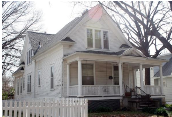
Sadly, this gable-front house at 517 South Sergeant Avenue burned in 2012 and will be demolished.
