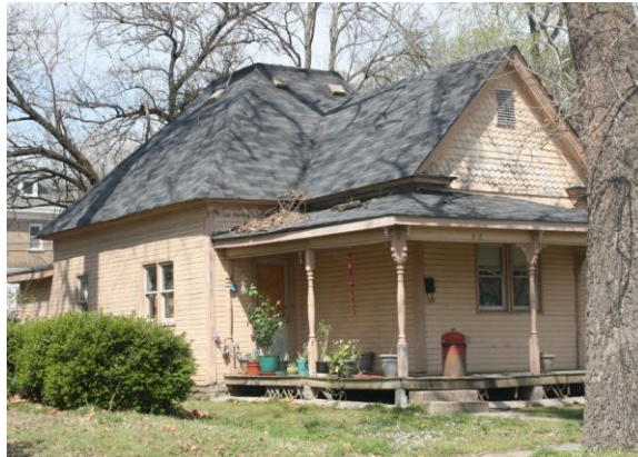
Modest c. 1890 cottage with an Eastlake-style wrap-around veranda
