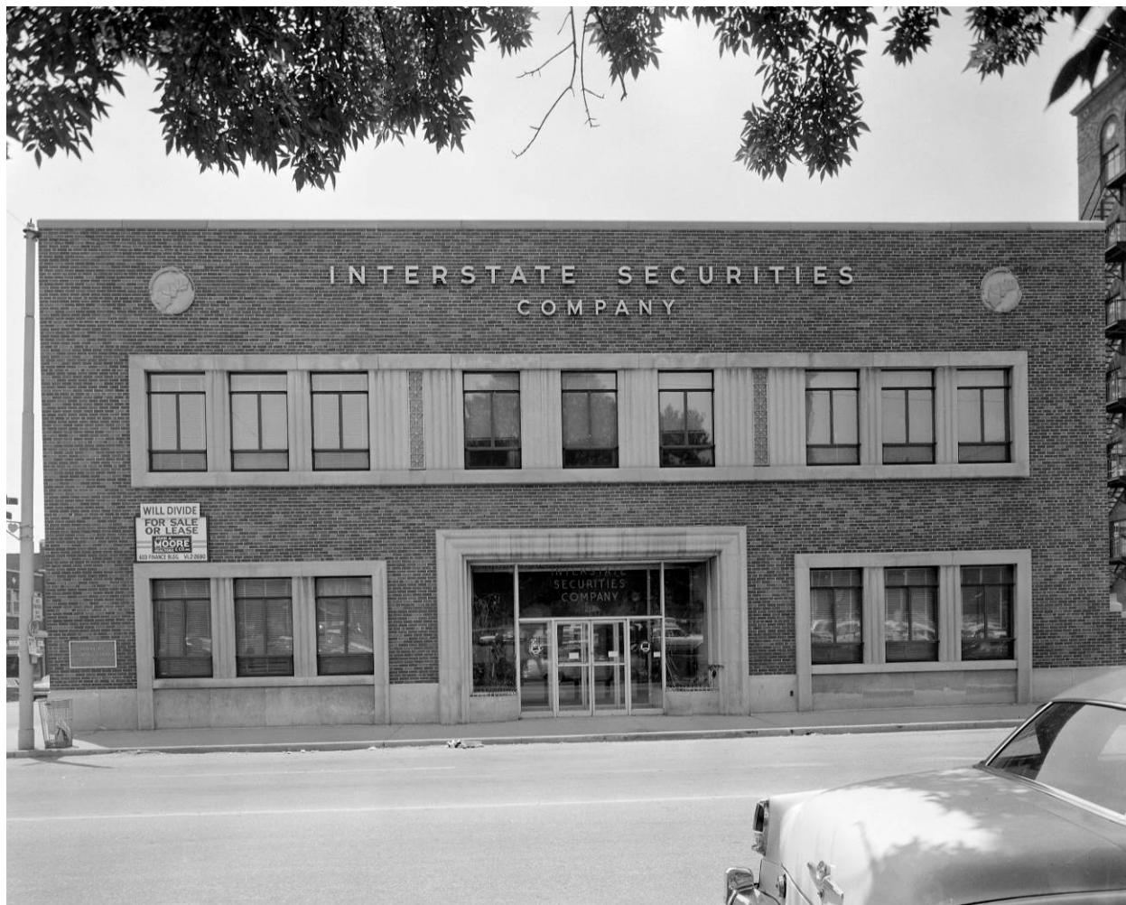
Figure 14. North elevation, c. 1962. Historic Photograph. Wilborn Photography, Kansas City, Missouri.
