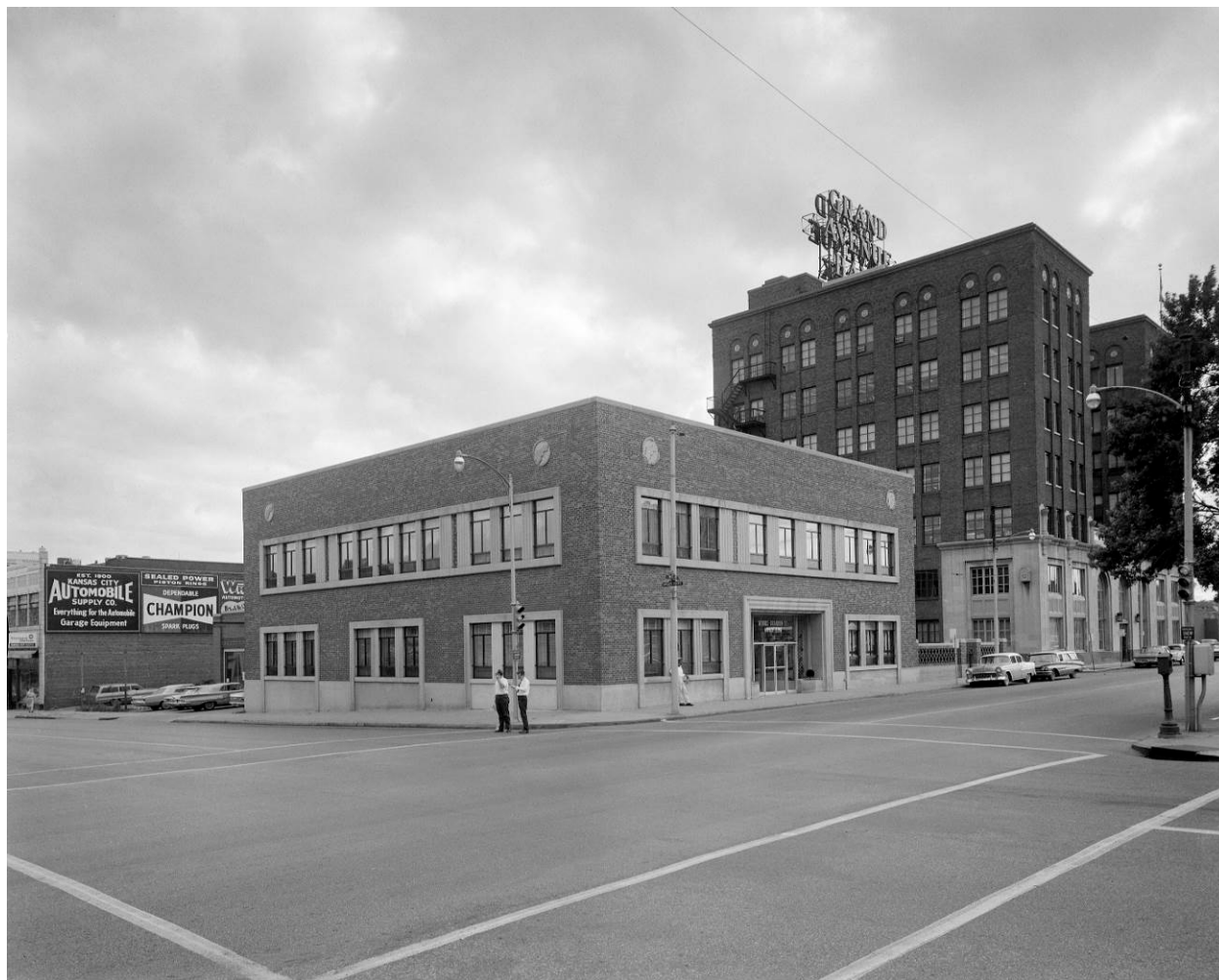
Figure 15. North and east elevations, c. 1964. Historic Photograph. Wilborn Photography, Kansas City, Missouri.
