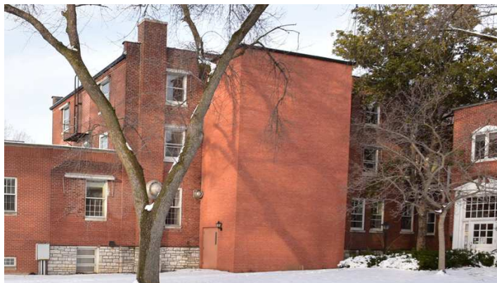
Figure 12: Resource 1, Block C, south elevation. Source: Brad Finch, F-Stop Photography, March 2015.
