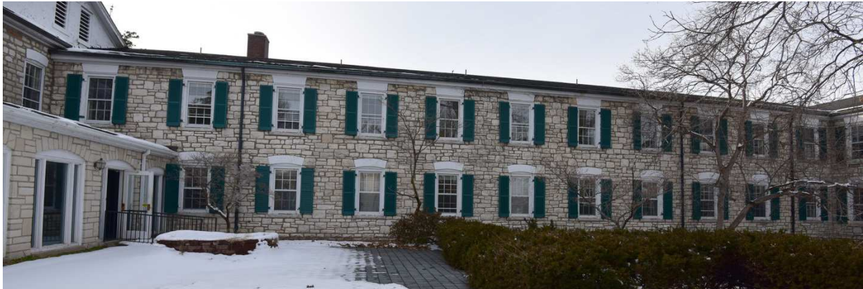
Figure 9: Resource 1, Block B, east elevation. Source: Brad Finch, F-Stop Photography, March 2015.
