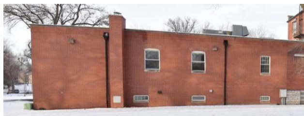
Figure 29: Resource 1, Block J, south elevation. Source: Brad Finch, F-Stop Photography, March 2015.
