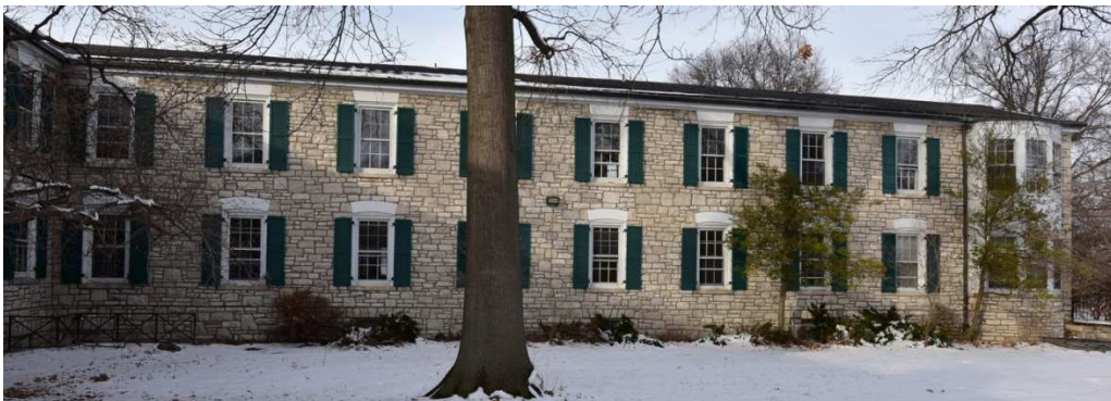
Figure 17: Resource 1, Block E, south elevation. Source: Brad Finch, F-Stop Photography, March 2015.
