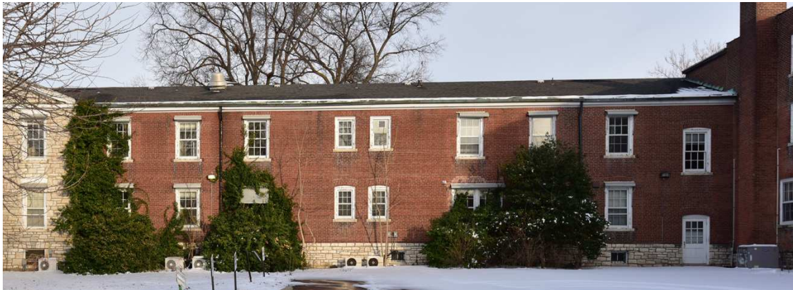
Figure 10: Resource 1, Block B, west elevation. Source: Brad Finch, F-Stop Photography, March 2015.
