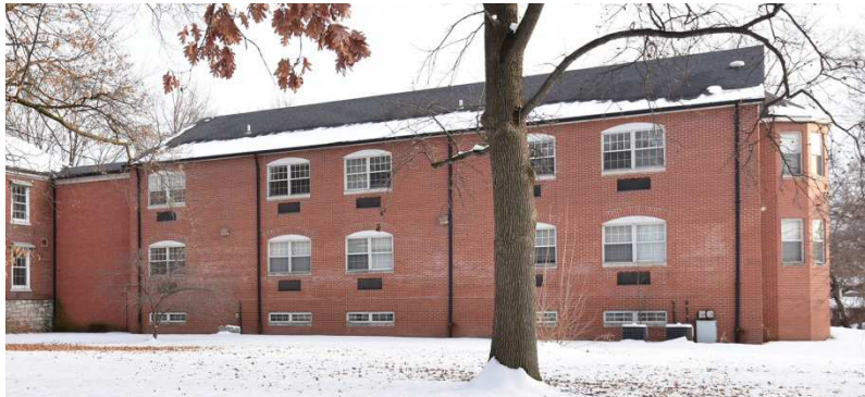
Figure 30: Resource 1, Block K, north elevation. Source: Brad Finch, F-Stop Photography, March 2015.
