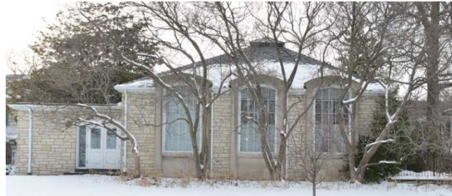
Figure 21: Resource 1, Block G, east elevation. Source: Brad Finch, F-Stop Photography, March 2015.
