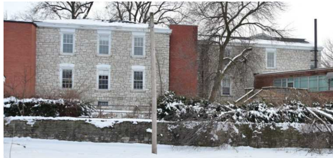
Figure 16: Resource 1, Block E, north elevation. Source: Brad Finch, F-Stop Photography, March 2015.
