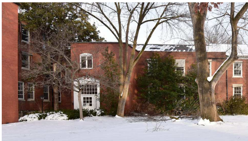
Figure 8: Resource 1, Block A, west elevation. Source: Brad Finch, F-Stop Photography, March 2015.
