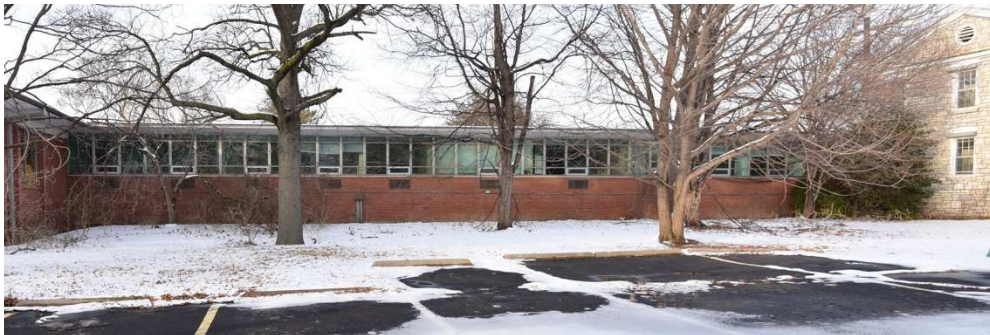
Figure 19: Resource 1, Block F, south elevation. Source: Brad Finch, F-Stop Photography , March 2015.
