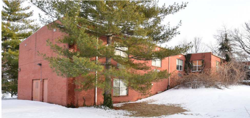
Figure 26: Resource 1, Block I, northwest corner. Source: Brad Finch, F-Stop Photography, March 2015.
