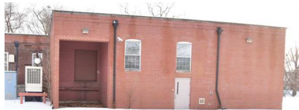
Figure 27: Resource 1, Block J, north elevation. Source: Brad Finch, F-Stop Photography, March 2015.
