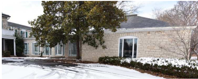
Figure 22: Resource 1, Block G, south elevation. Source: Brad Finch, F-Stop Photography, March 2015.
