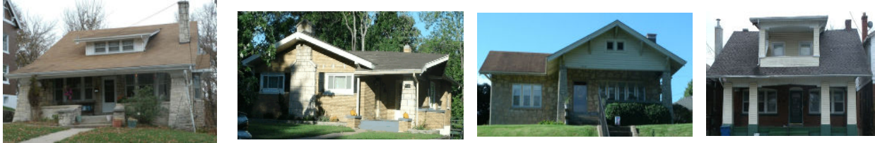
Figure 12. Bungalows exhibiting battered columns in Jefferson City 508 Jackson, left, is one of a very few Bungalows in Jefferson City with battered columns and a shed roof. Other examples with battered columns are 930 Fairmount, 1903 W. Main and 817 Clark Avenue.
